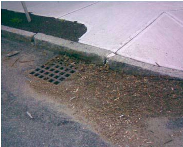
Figure 2-16 Deep sump catch basin inlet
