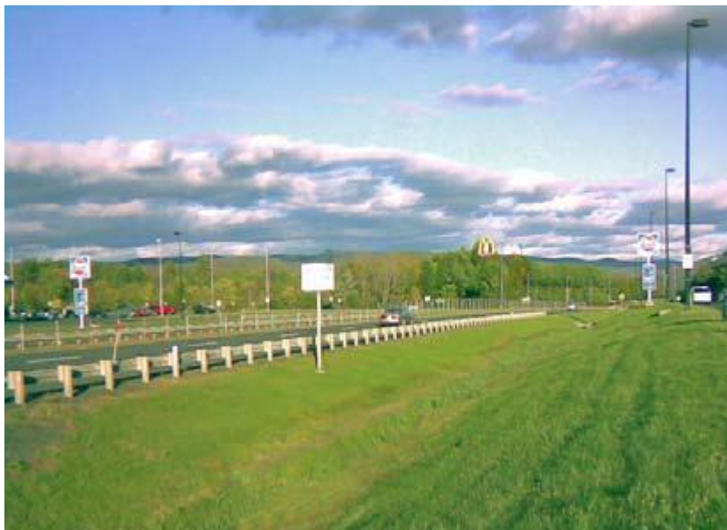
Figure 2-1 Dry water quality swale
