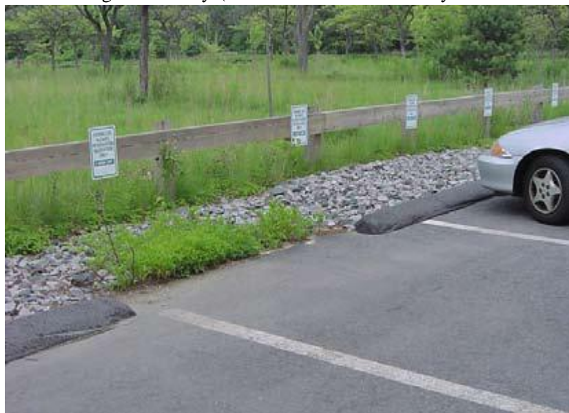
Figure 2-3 Vegetated filter strip
