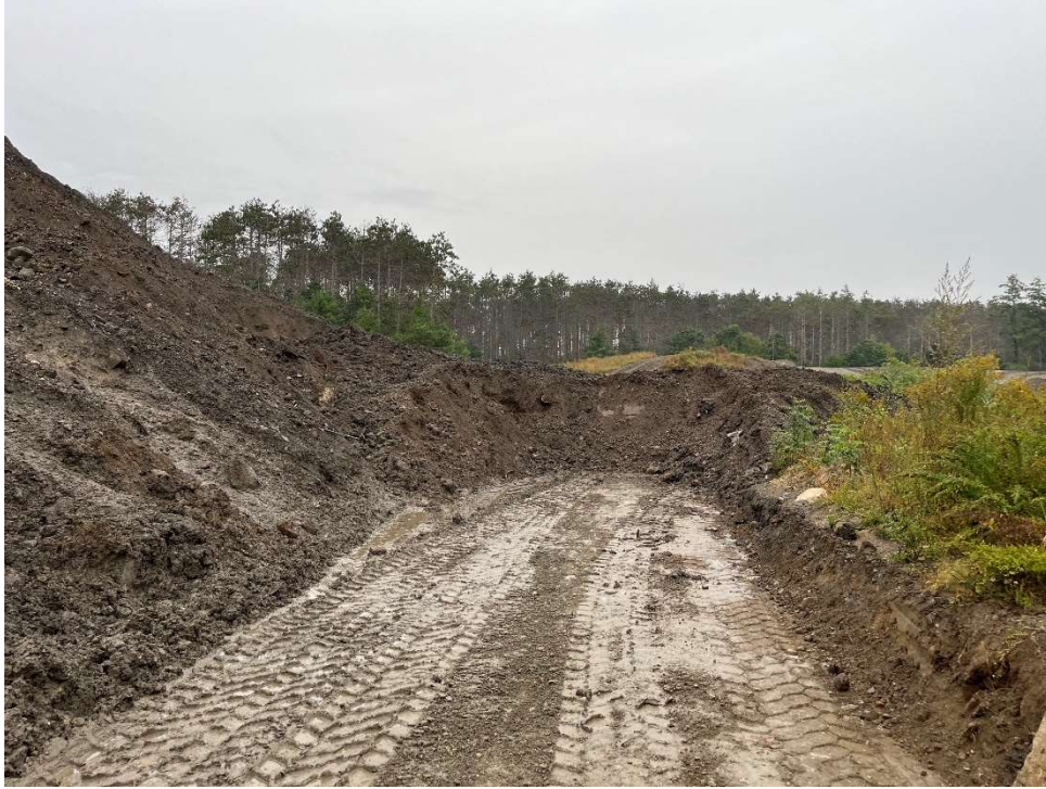
Photo 7 – Fill material placed over previous access road
