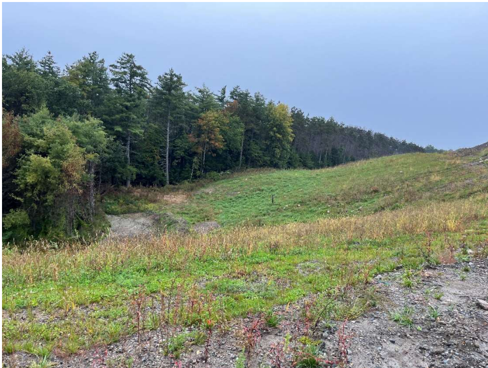
Photo 6 – Monitoring well and southwestern slope.
