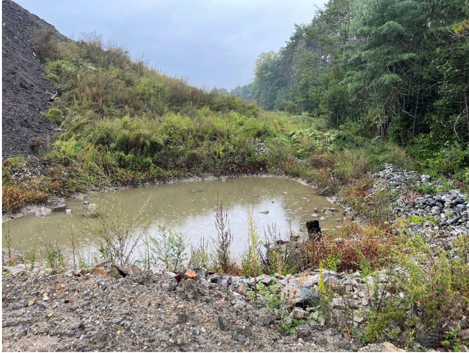
Photo 9 - Temporary rip rap settling area.
