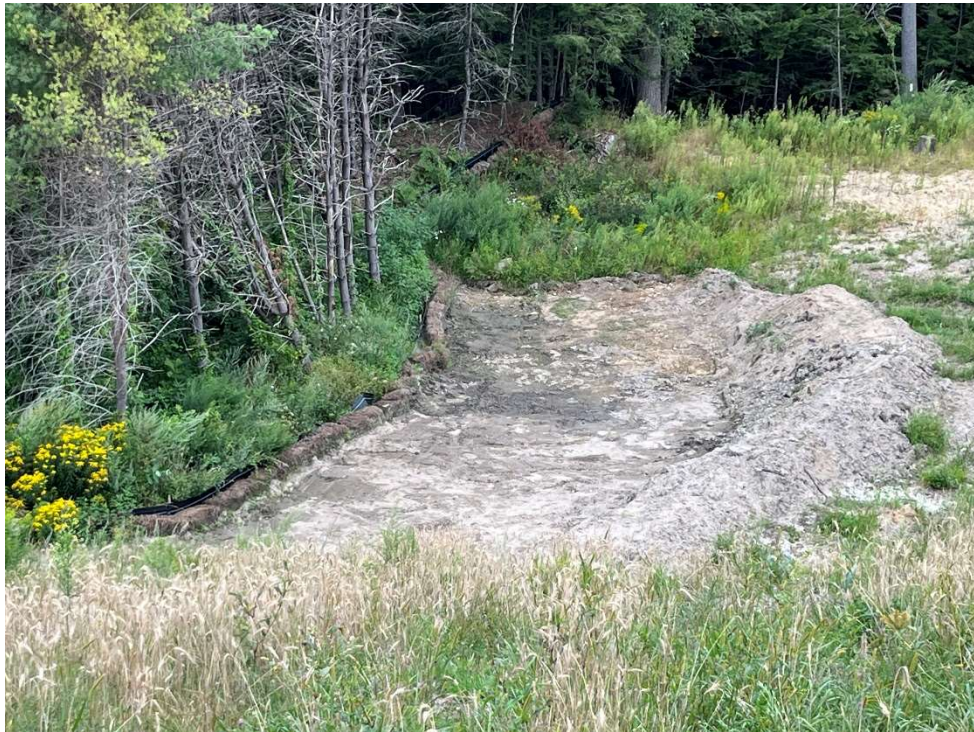
Photo 4 – Southwestern slope with sediment cleared from against the erosion control.
