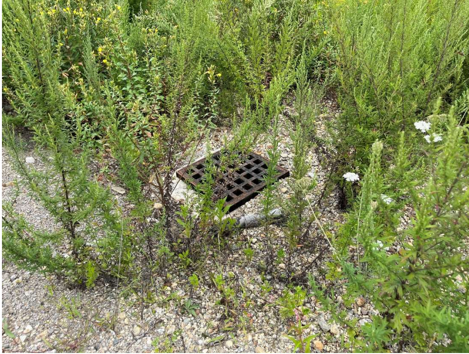
Photo 7 – Temporary stormwater overflow catch basin.
