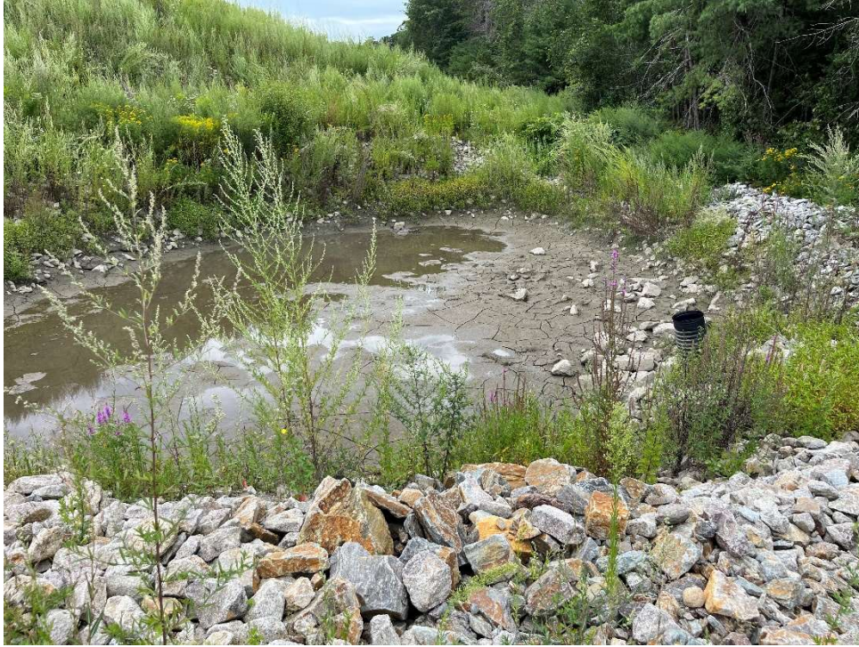
Photo 9 - Temporary rip rap settling area.
