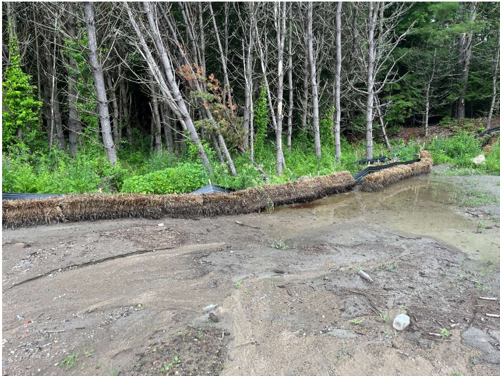
Photo 4 – Southwestern slope with sediment and water accumulating against the erosion control.
