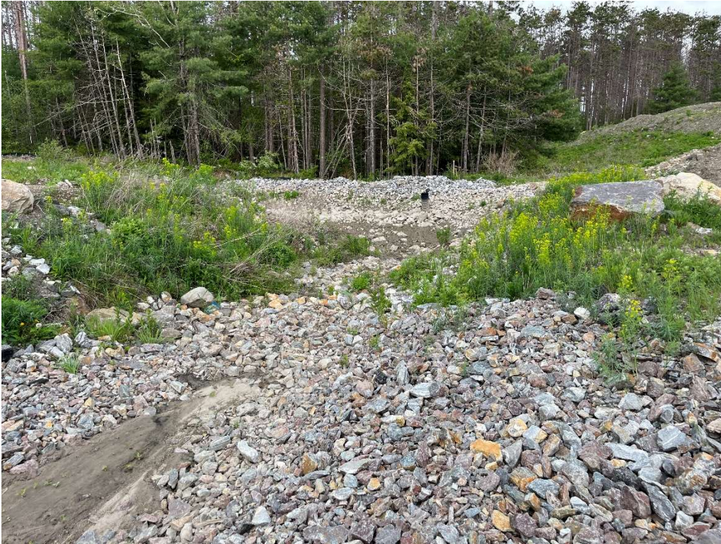
Photo 9 - Temporary rip rap settling area.
