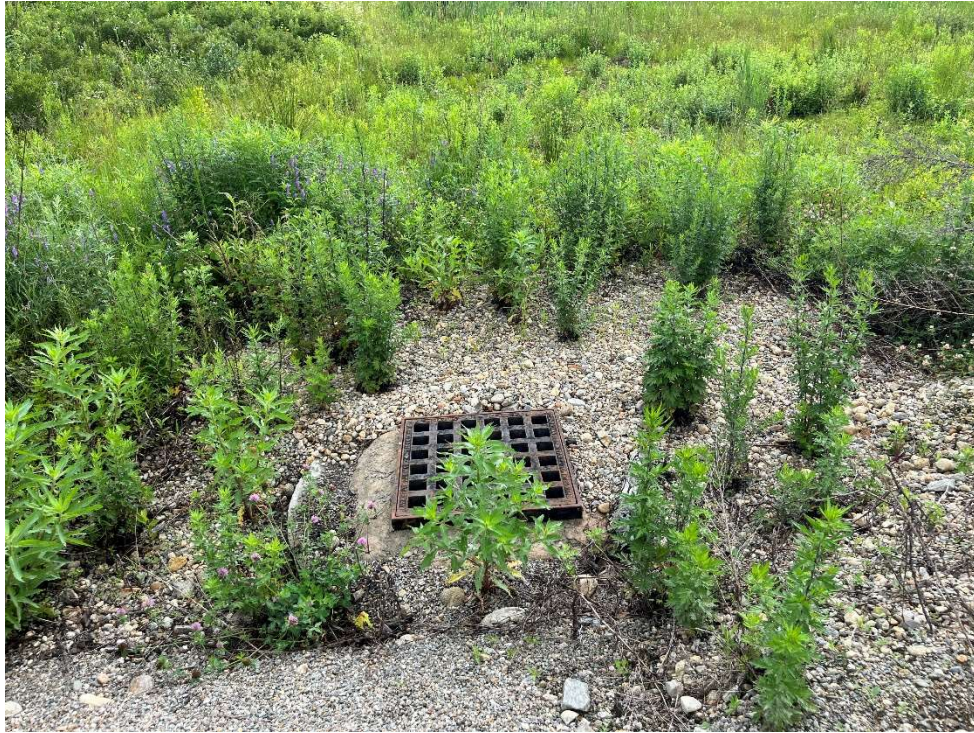
Photo 7 – Temporary stormwater overflow catch basin.
