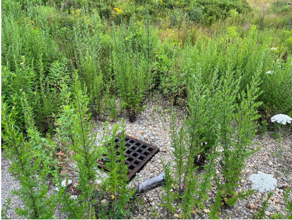
Photo 7 – Temporary stormwater overflow catch basin.
