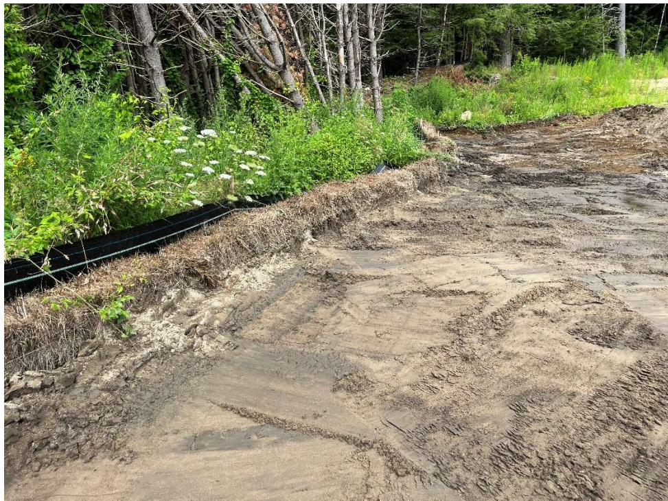
Photo 4 – Southwestern slope with sediment accumulating against the erosion control.
