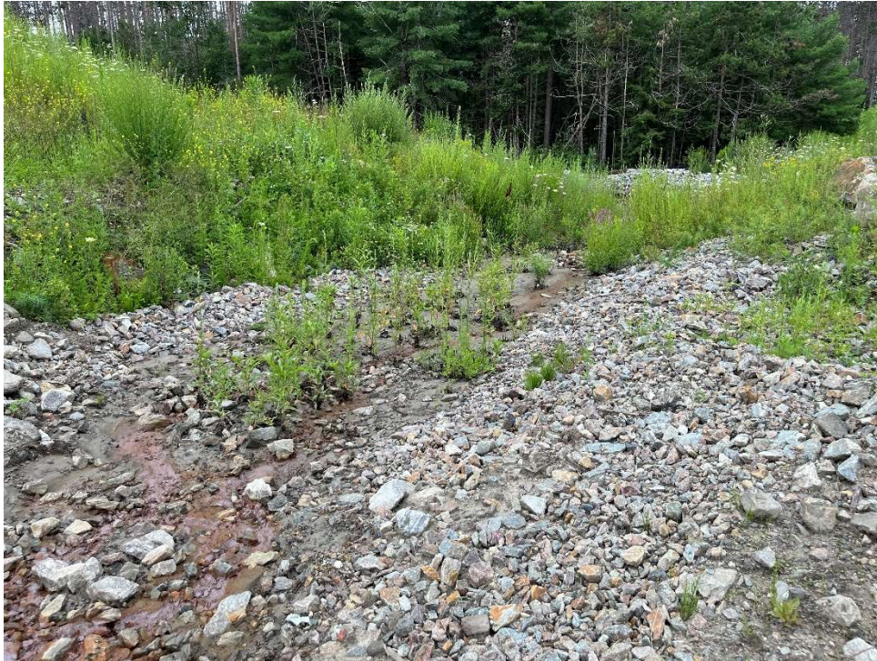
Photo 9 - Temporary rip rap settling area.
