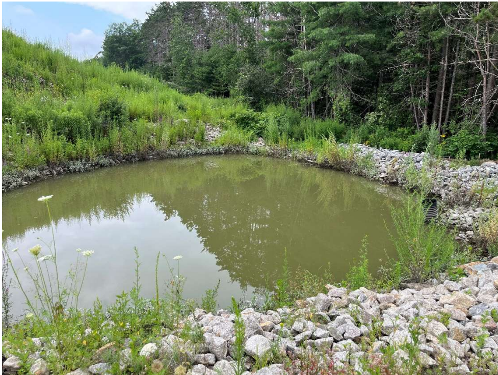
Photo 8 – Swale between temporary stormwater basin and temporary rip rap settling area.
