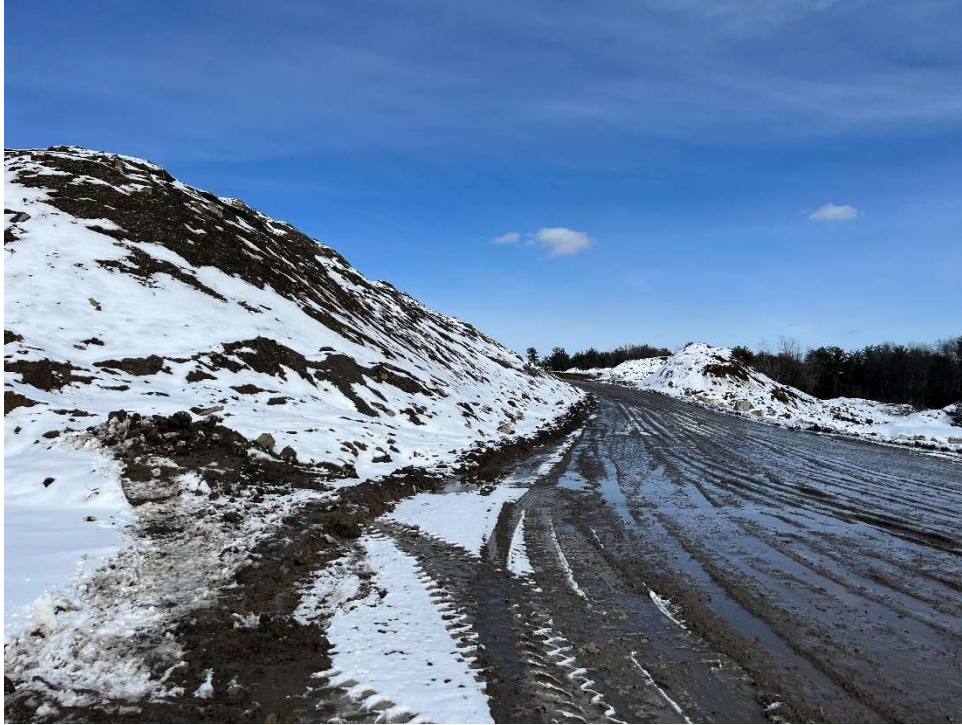
Photo 13 –Material placed and graded at the center of the Site with grading for truck access
