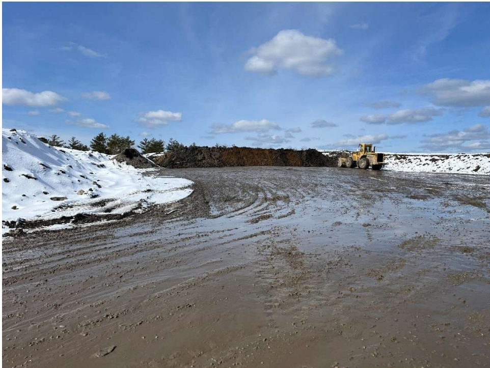
Photo 14 –Material placed and graded at the center of the Site with grading for truck access
