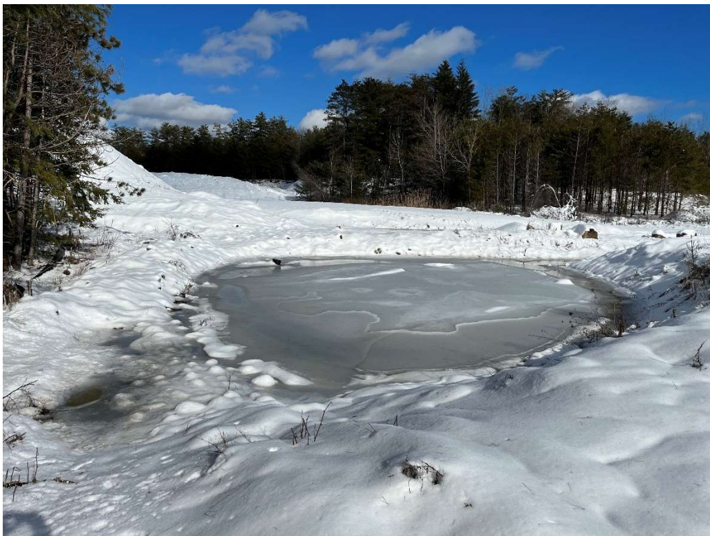
Photo 10 - Temporary rip rap settling area.
