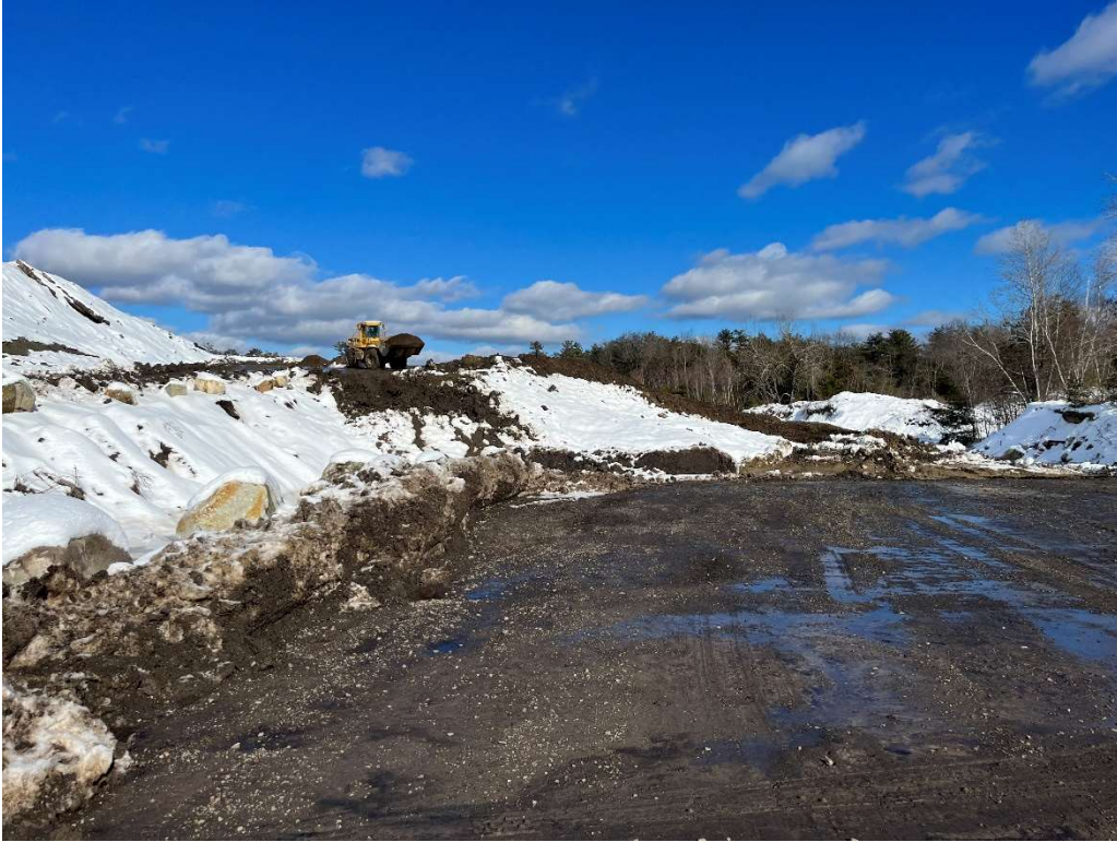
Photo 1 – Eastern slope and access road, looking north.
