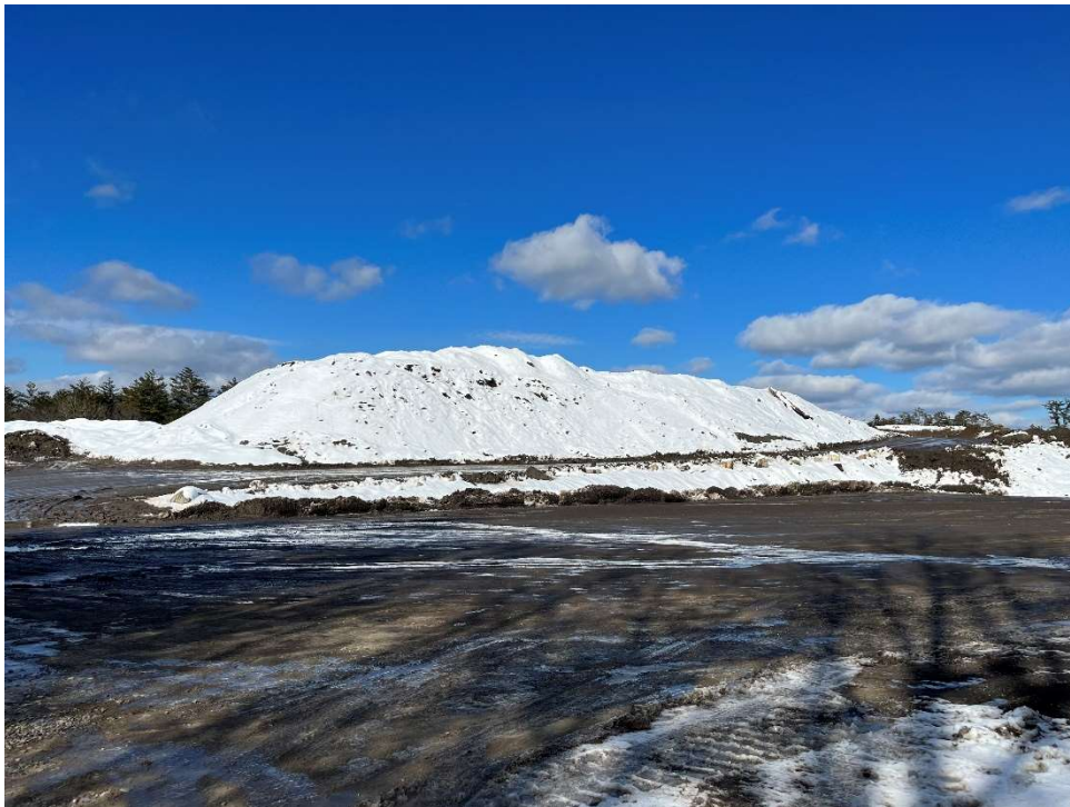
Photo 4 –Material placed and graded at the center of the Site with grading for truck access
