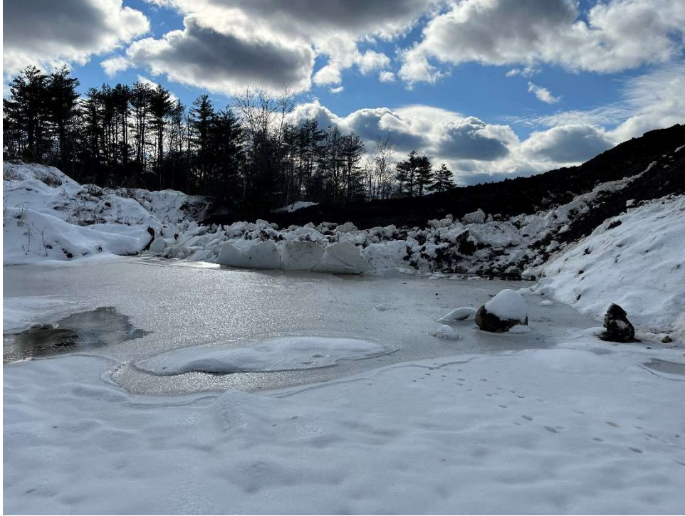
Photo 3 –Fill placed over location of previous access road
