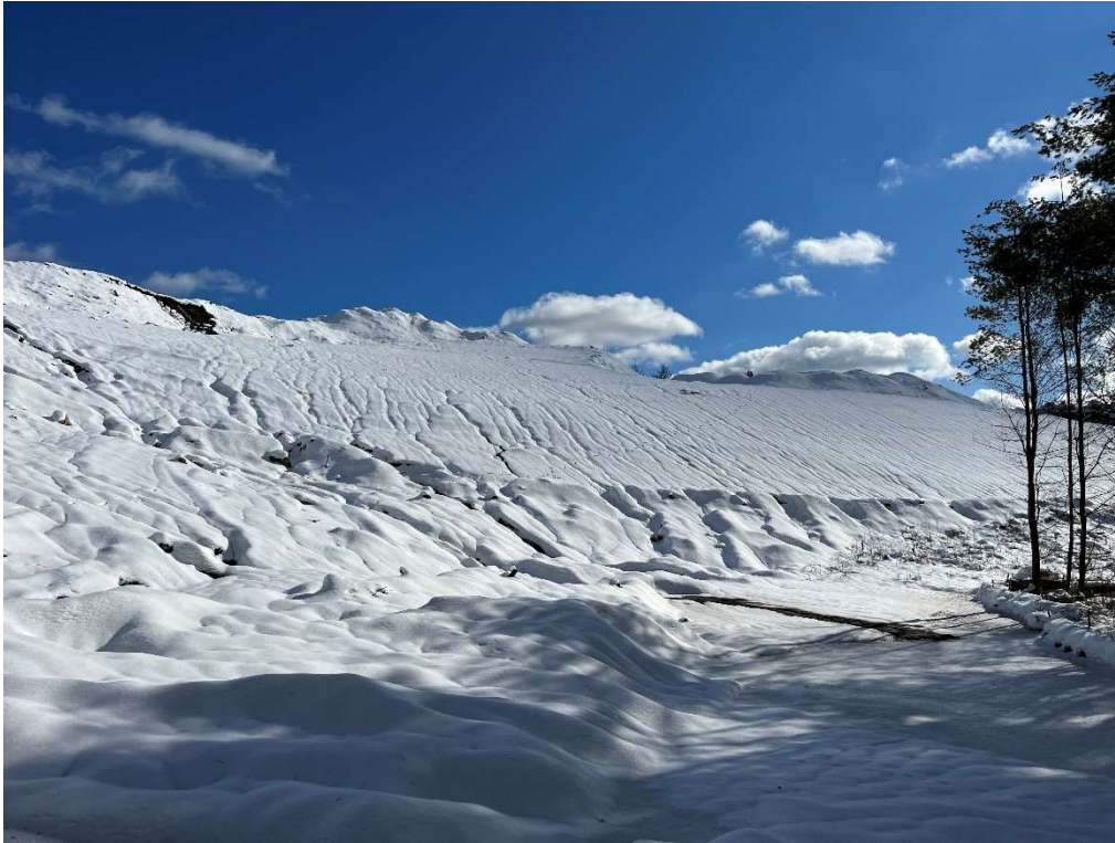
Photo 5 – Southwestern slope with erosion and standing water.
