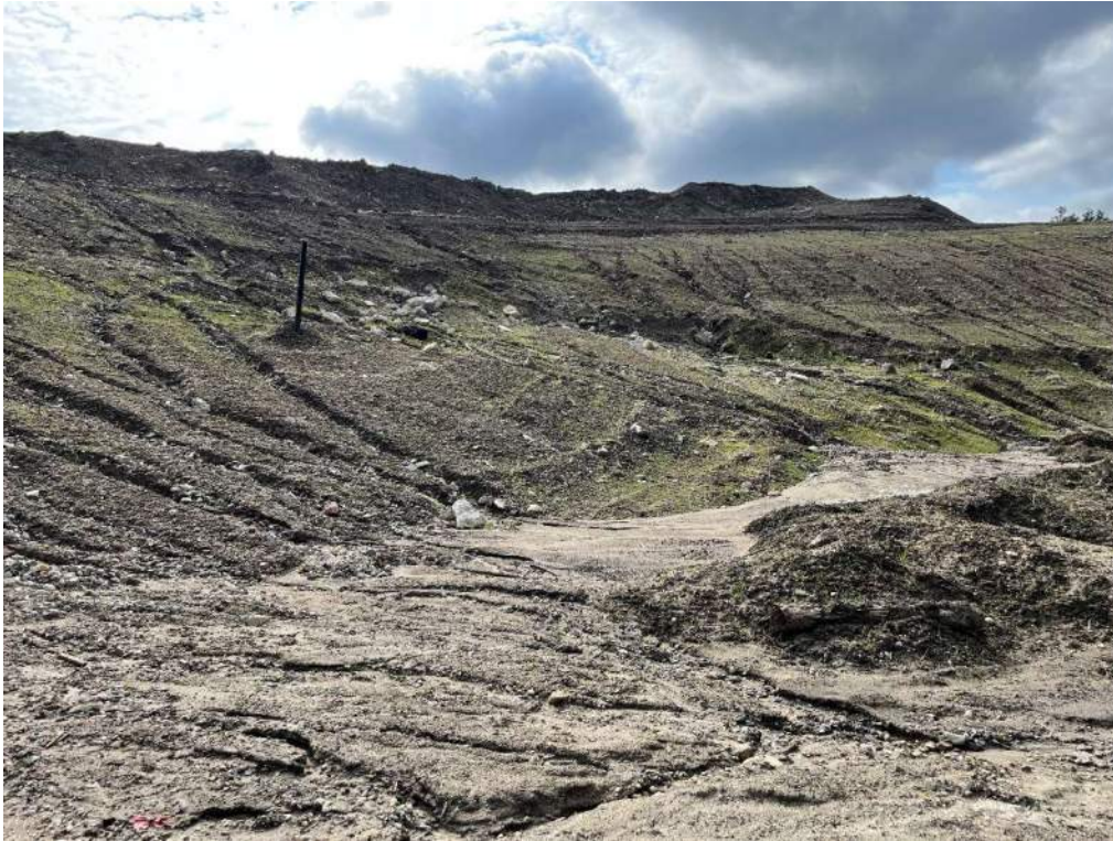
Photo 5 – Monitoring well and erosion in the southwestern slope.
