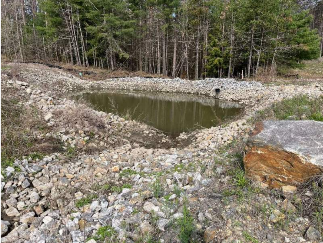
Photo 9 - Temporary rip rap settling area.
