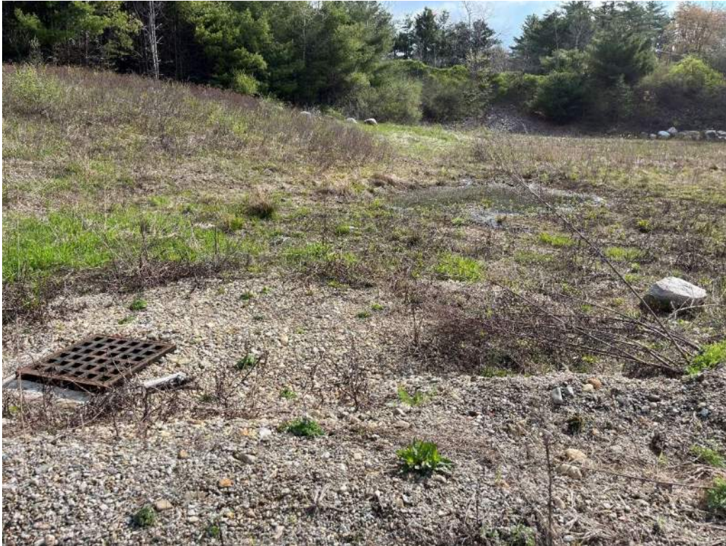
Photo 7 – Temporary stormwater overflow catch basin.
