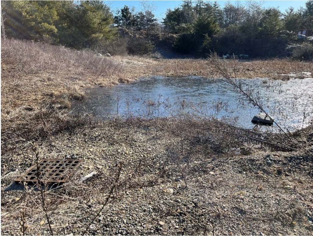
Photo 9 – Temporary stormwater overflow catch basin.
