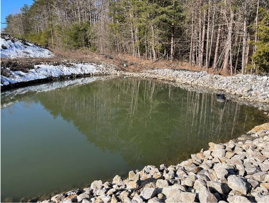
Photo 11 - Temporary rip rap settling area.
