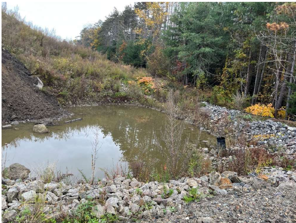
Photo 8 - Temporary rip rap settling area.
