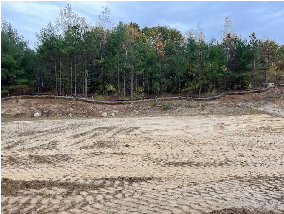
Photo 6 – Erosion control placed on the east edge of the site
