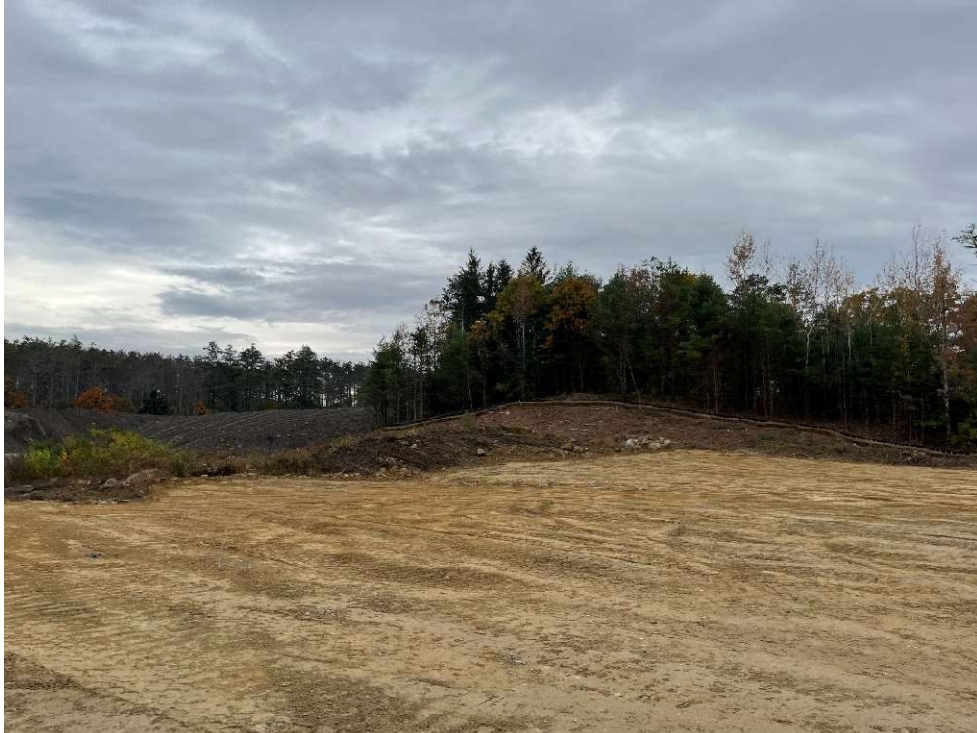
Photo 7 – Grading and shaping material placed in the area of the proposed north stormwater basin
