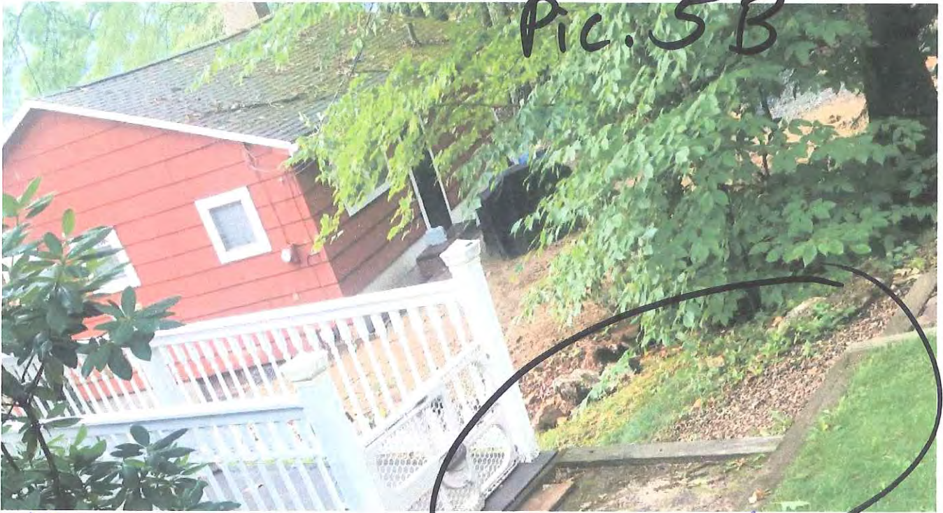
Platform connecting side entrance + front walkway.
