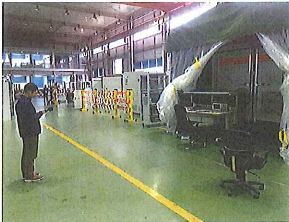
5m away from Inverter
