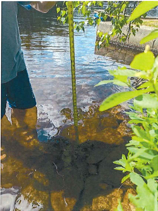
Figure 4. Summer photo taken near north end of restored stone wall. Stone wall will tie into 3 ft concrete wall to north.
