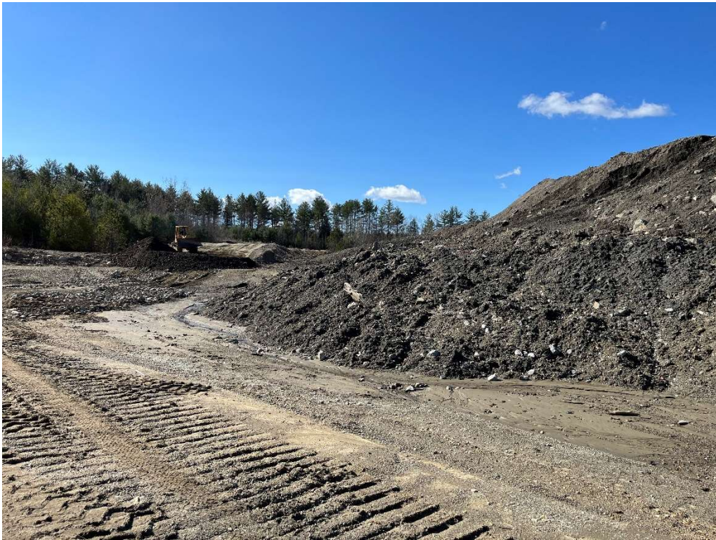
Photo 3 – Eastern slope and construction of new access road.
