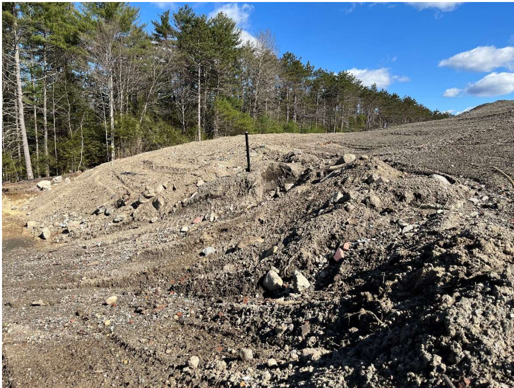
Photo 10 – Grading at monitoring well.
