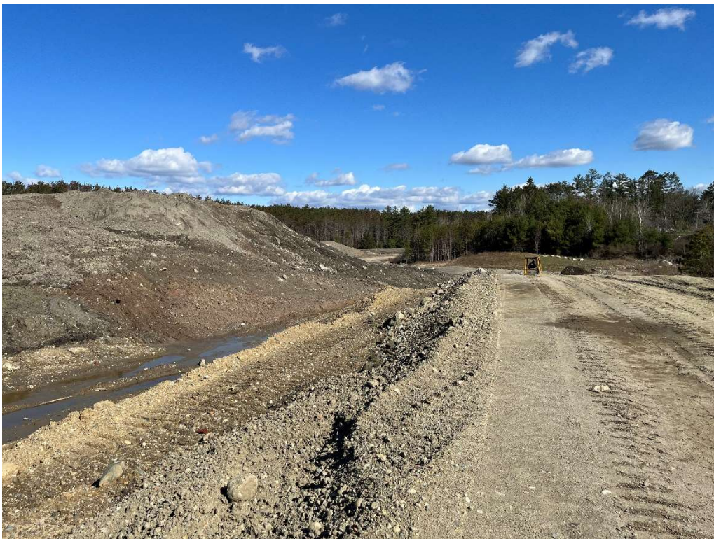
Photo 2 – Eastern slope and construction of new access road.
