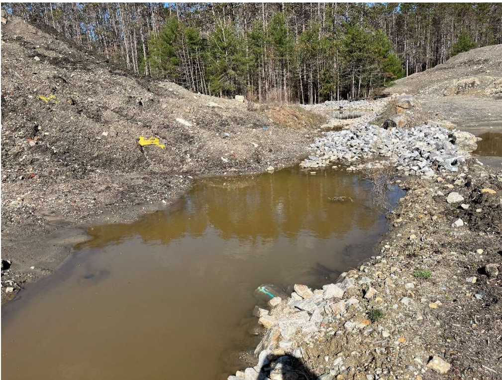
Photo 6 – Swale between temporary stormwater basin and temporary rip rap settling area.
