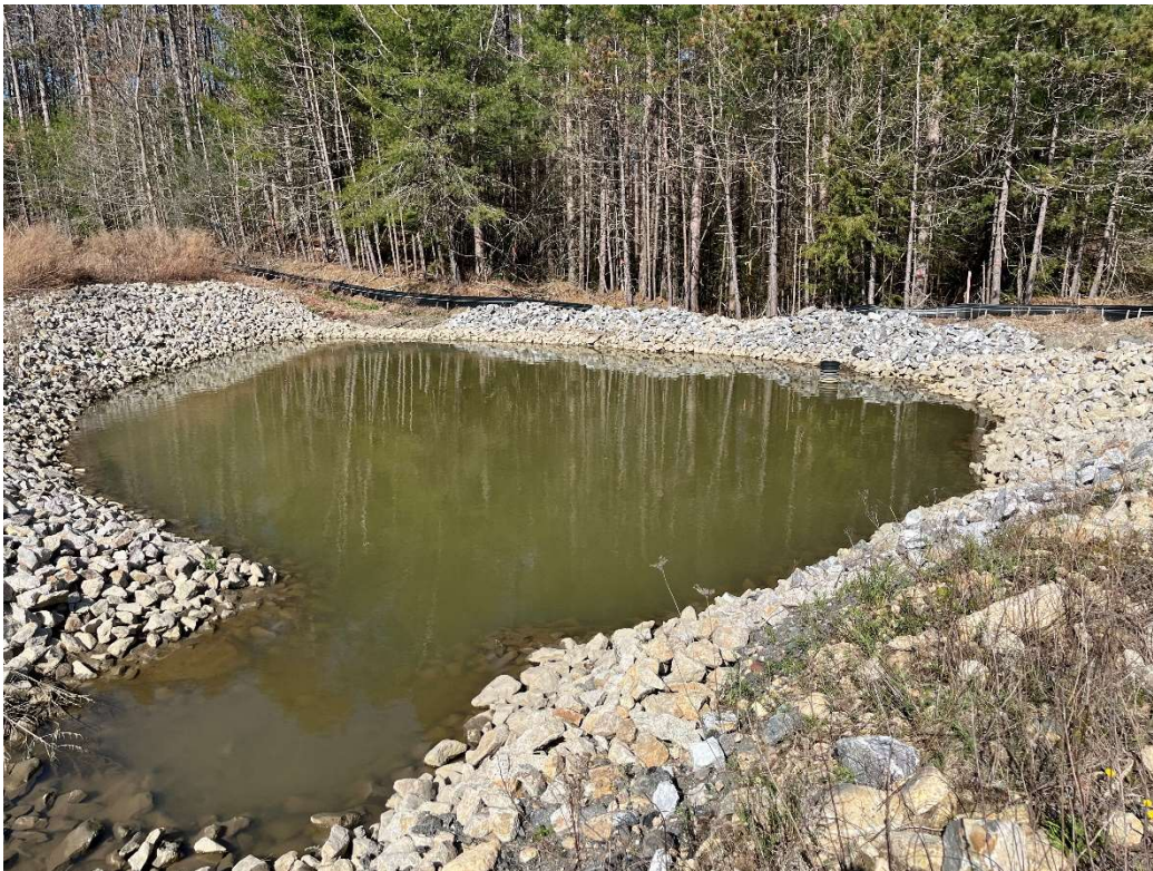
Photo 7 - Temporary rip rap settling area.
