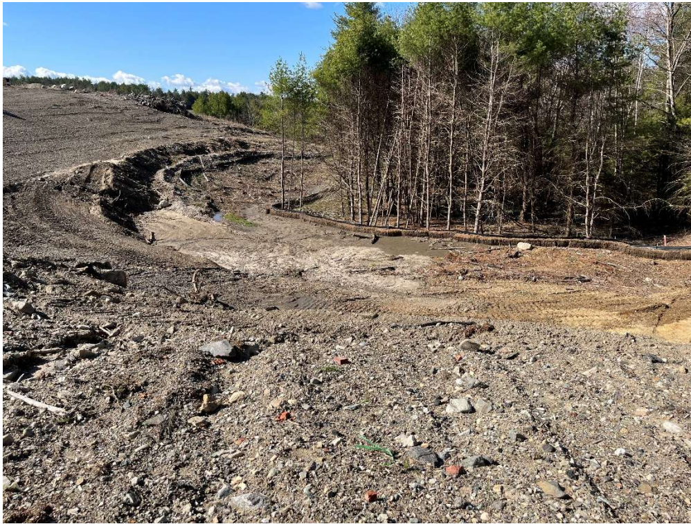
Photo 9 – Southwestern slope and erosion control.
