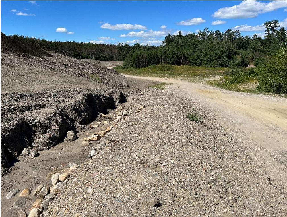
Photo 3 – Eastern slope, temporary swale, and access road.
