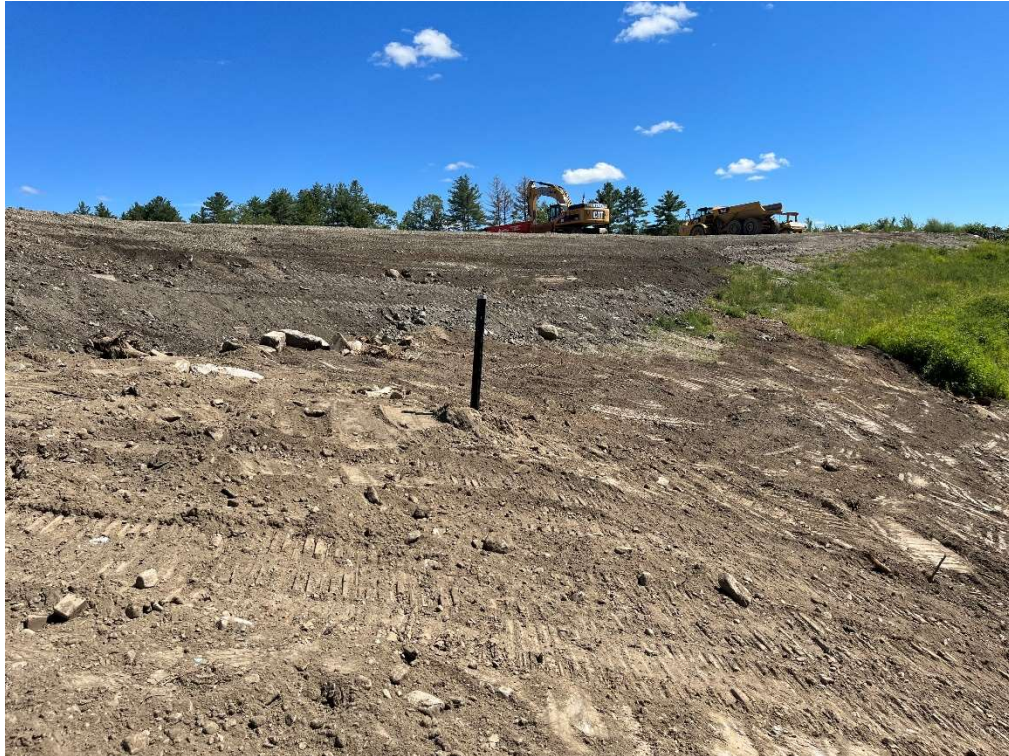
Photo 11 – Grading at monitoring well.
