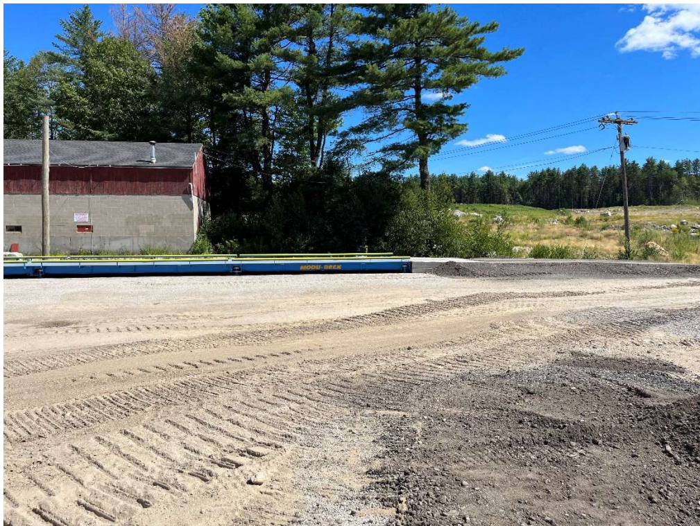
Photo 12 – New scale and concrete pad
