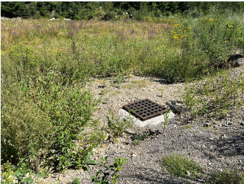
Photo 4 – Temporary stormwater overflow catch basin.
