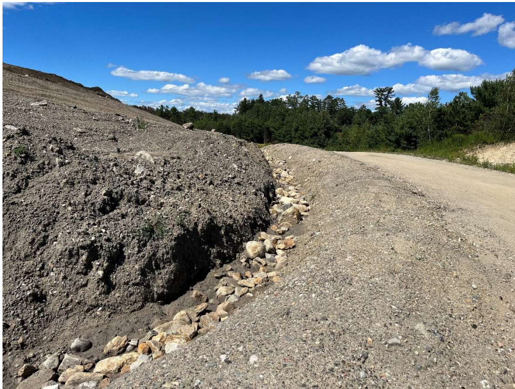
Photo 2 – Temporary swale and access road.
