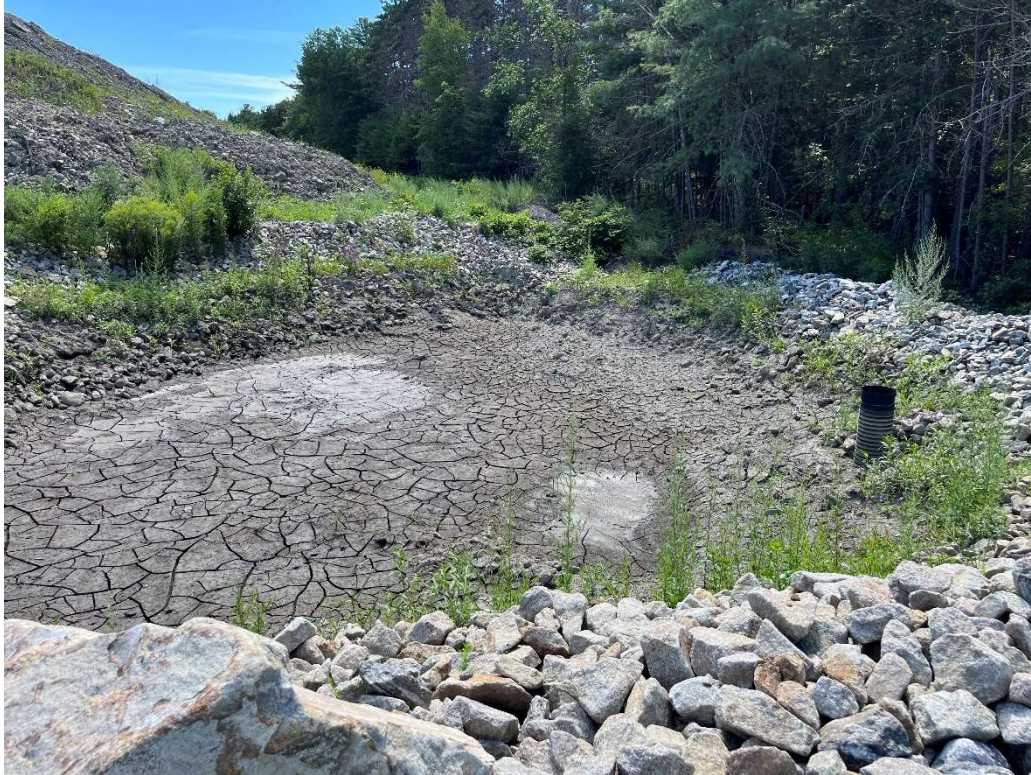
Photo 7 - Temporary rip rap settling area.
