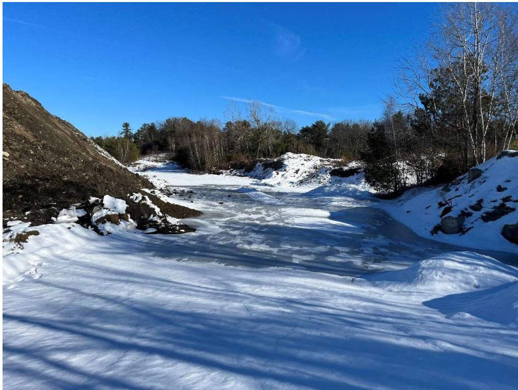
Photo 2 – Eastern slope and damaged access road, looking north.
