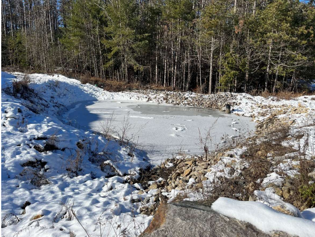
Photo 9 - Temporary rip rap settling area.
