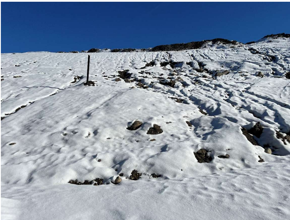
Photo 6 – Monitoring well and erosion in the southwestern slope.
