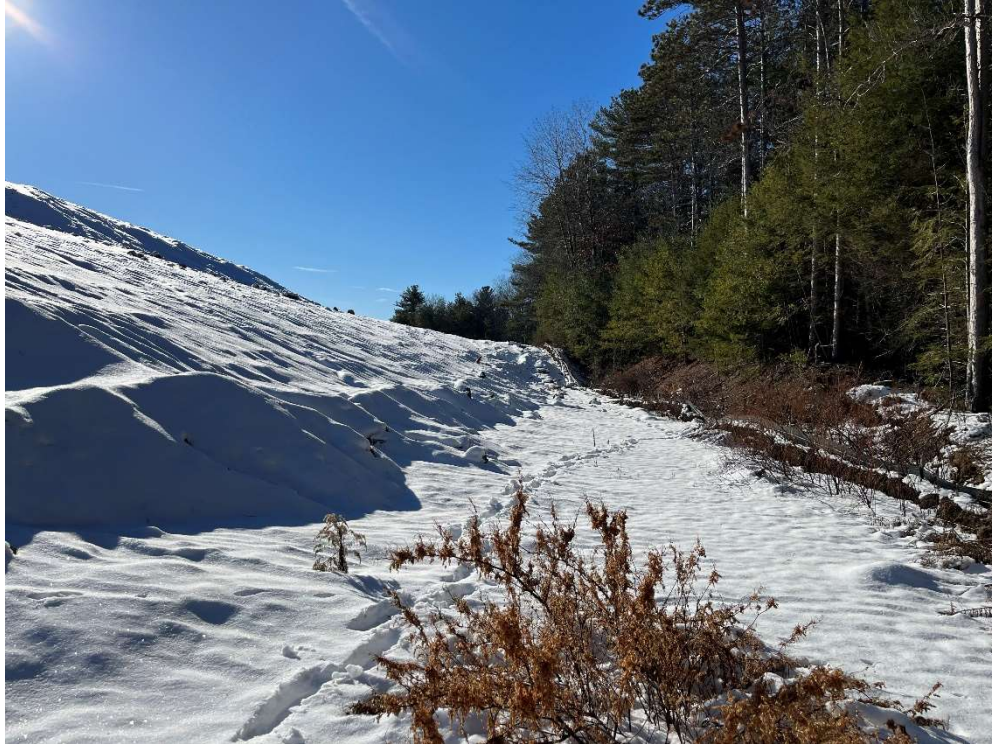
Photo 11 –Erosion control with sediment buildup on the western limits of the Site.
