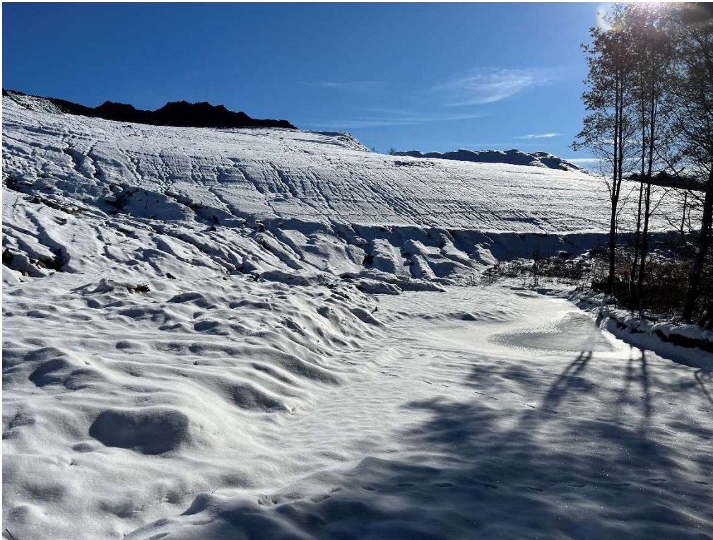
Photo 4 – Southwestern slope with erosion and standing water.
