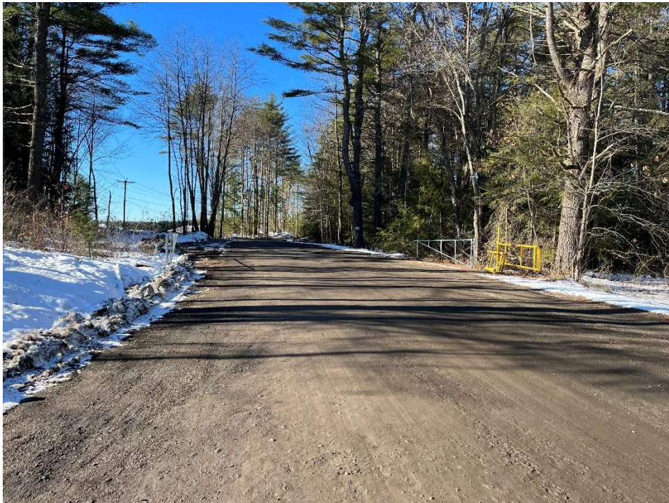
Photo 14 – New gate at access road entrance from River
