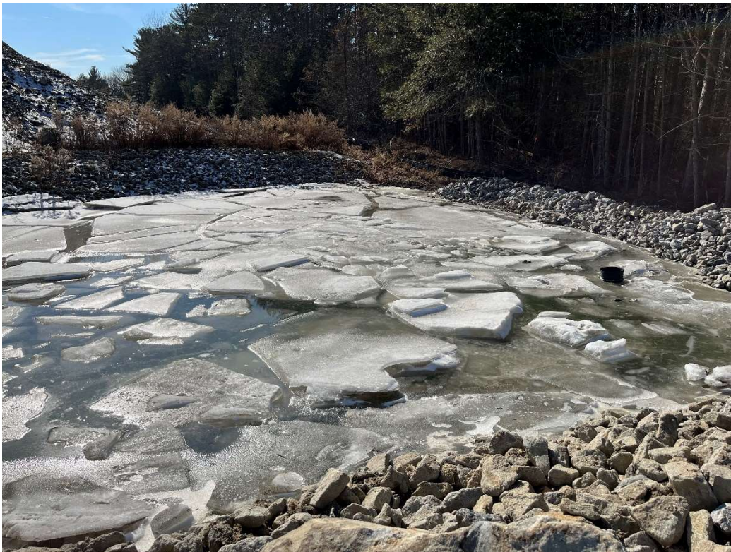
Photo 5 - Temporary rip rap settling area.
