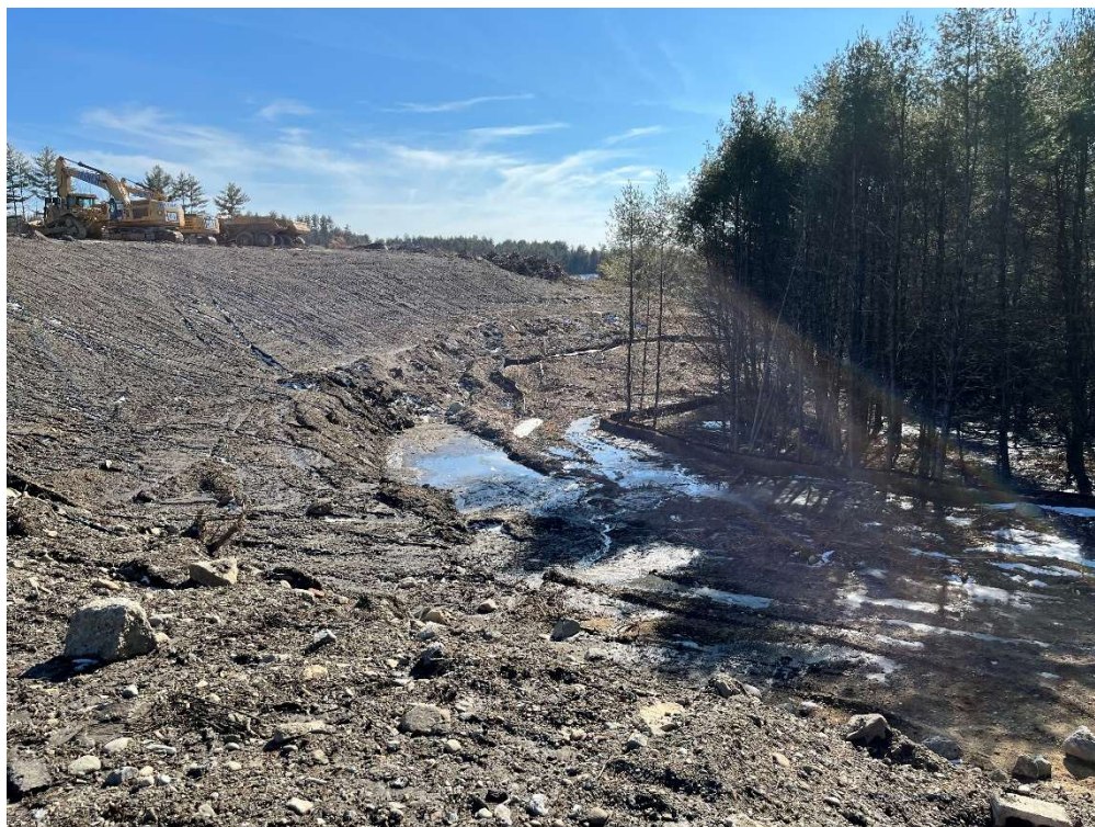
Photo 8 – Southwestern slope and erosion control.
