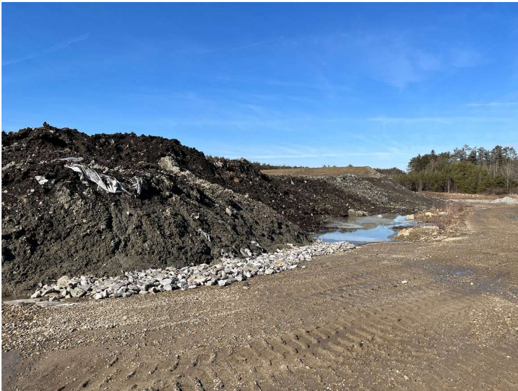
Photo 1 – Eastern slope and access road.
