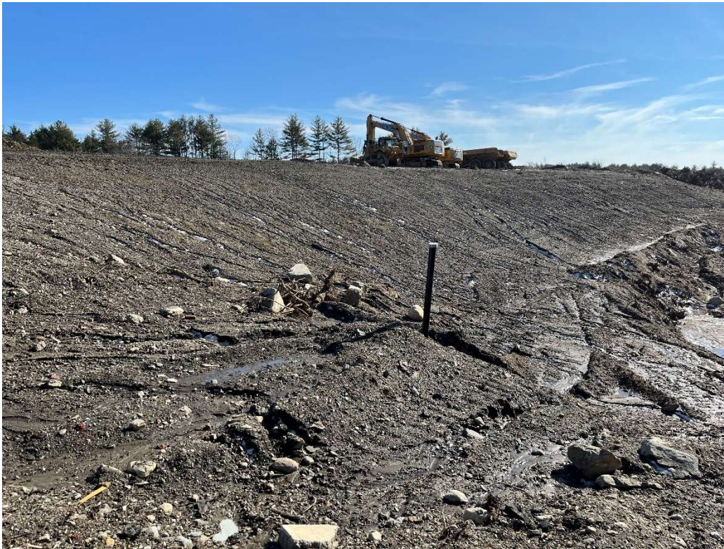
Photo 9 – Grading at monitoring well.
