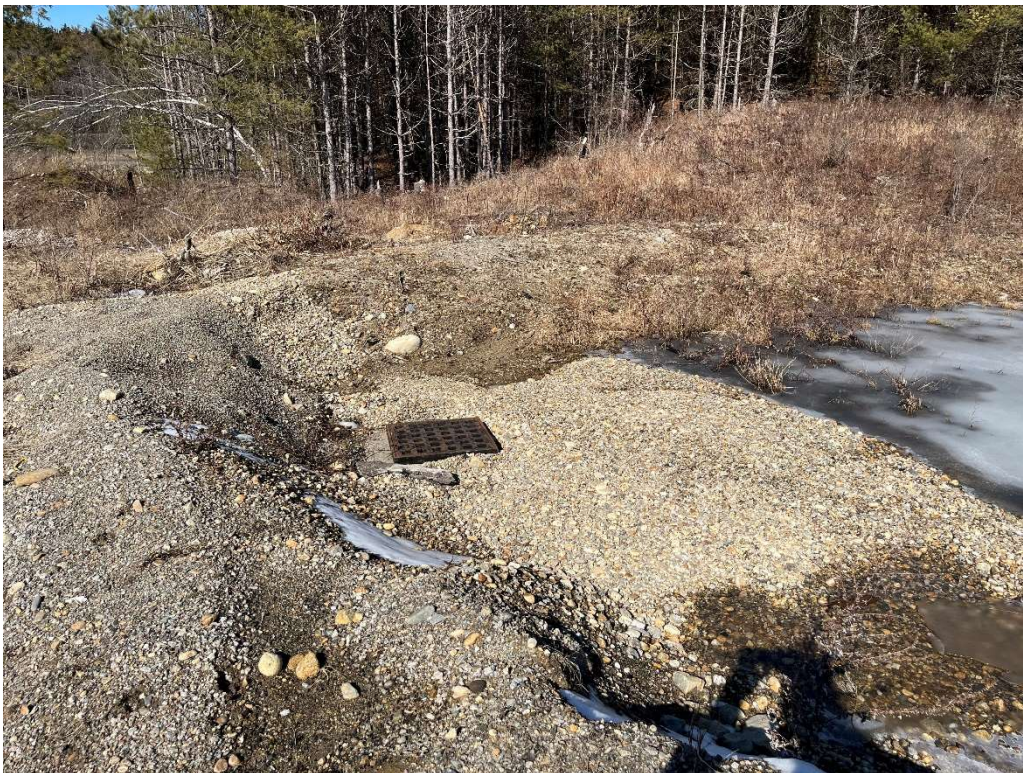
Photo 2 – Temporary stormwater overflow catch basin.
