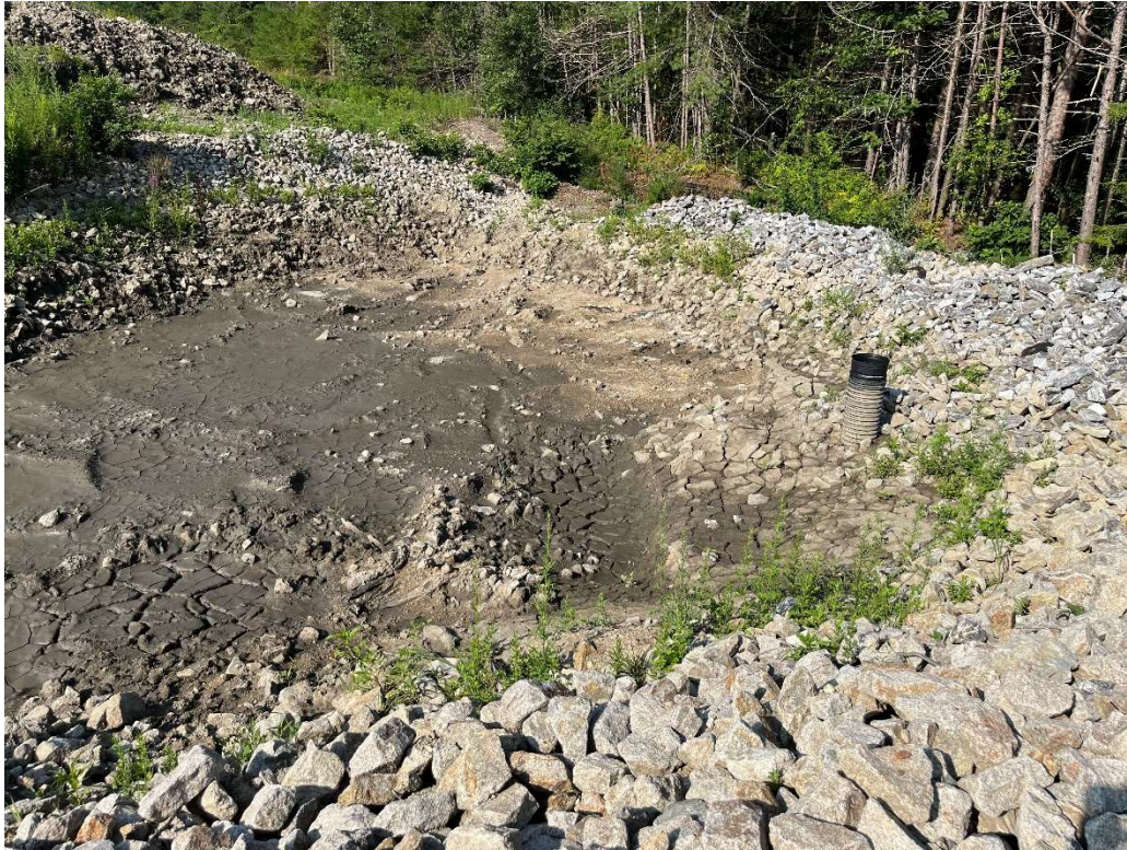
Photo 7 - Temporary rip rap settling area.
