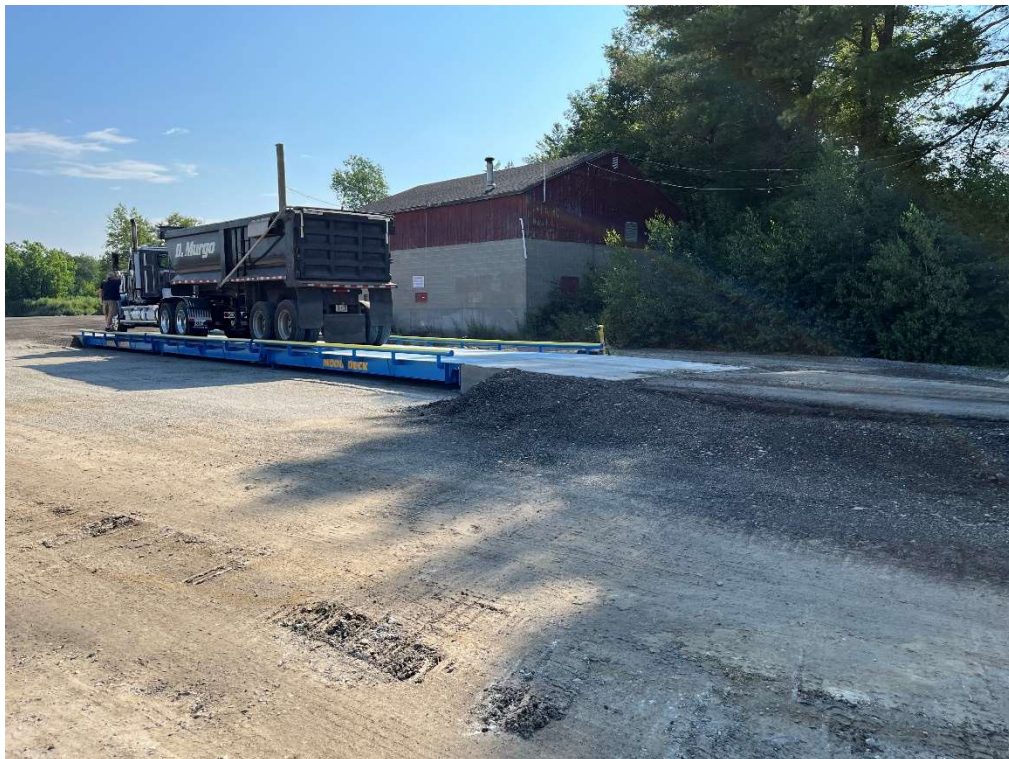
Photo 12 – New scale and concrete pads
