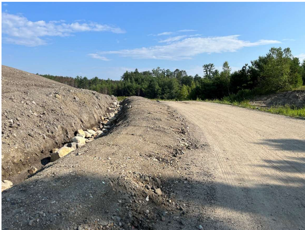
Photo 2 – Temporary swale and access road.
