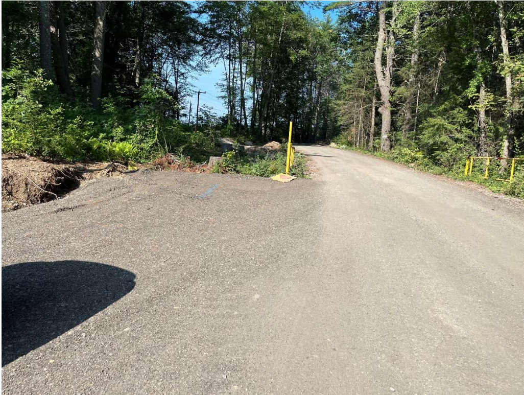
Photo 15 – Expanded access road and River Street entrance.
