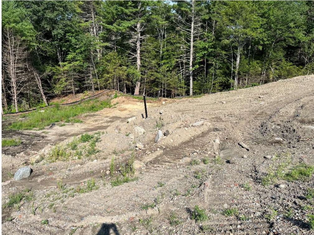
Photo 11 – Grading at monitoring well.
