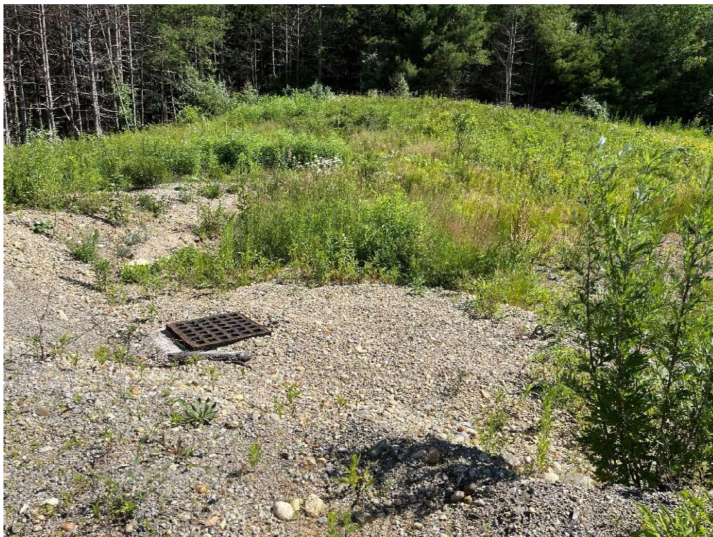
Photo 4 – Temporary stormwater overflow catch basin.
