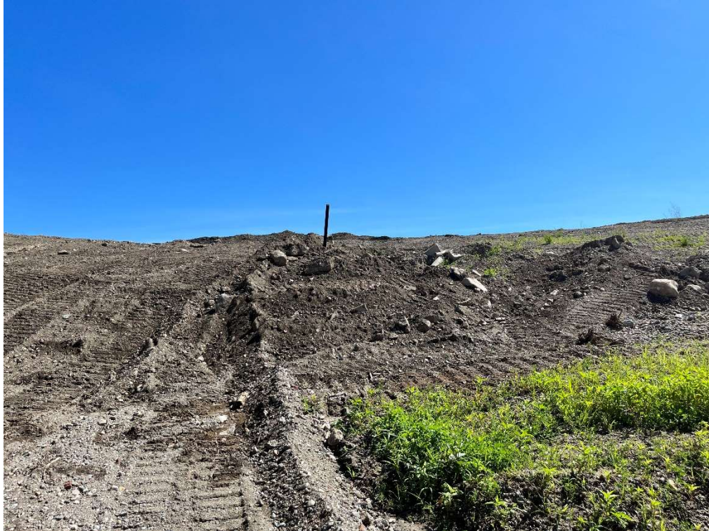
Photo 11 – Grading at monitoring well.
