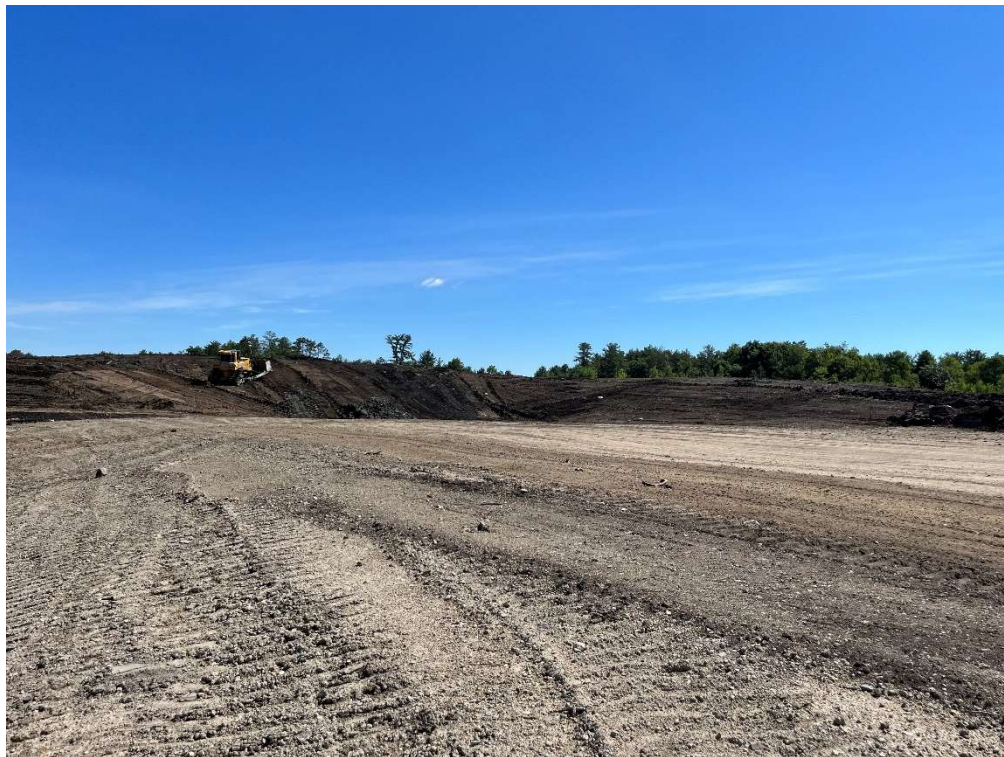
Photo 10 – Material placed for grading and shaping.
