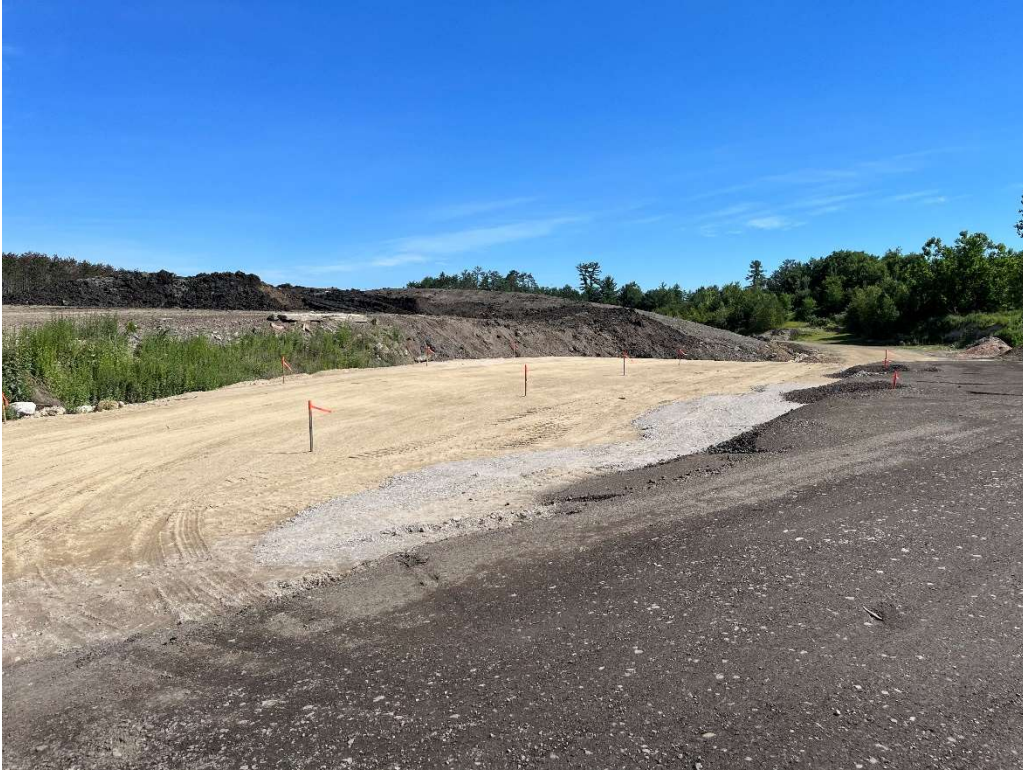
Photo 1 – Eastern slope and access road.
