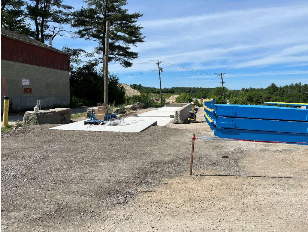
Photo 13 – Concrete pad for new scale.
