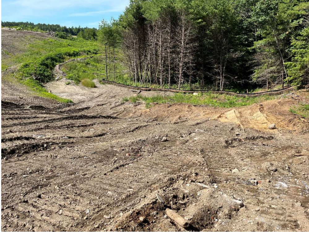
Photo 9 – Slope and erosion control at southwestern limits of the Site.
