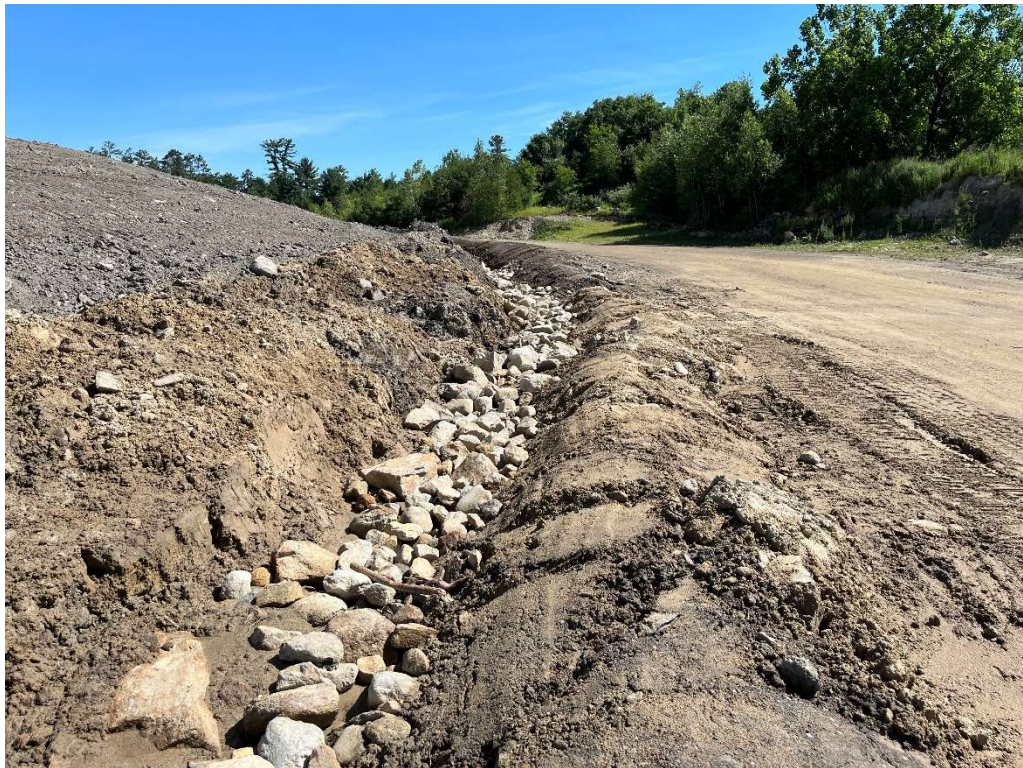
Photo 2 – Temporary swale and access road.
