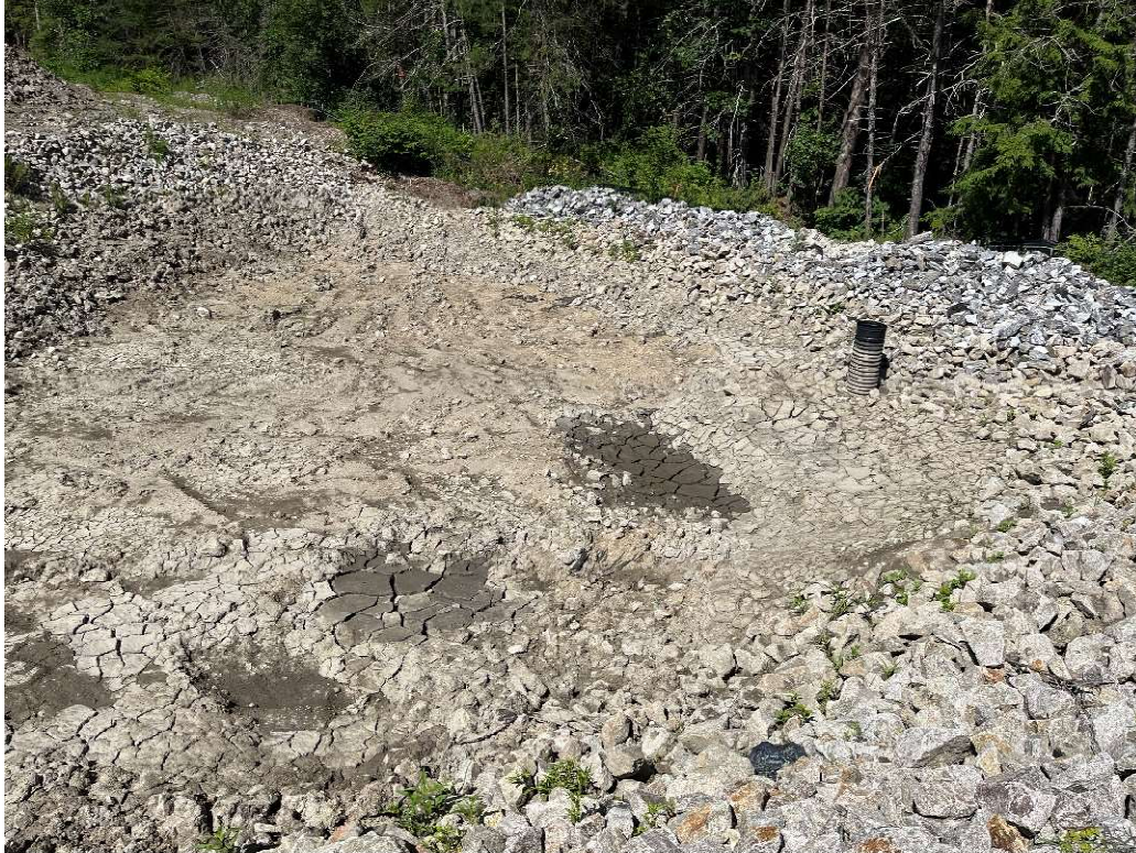
Photo 7 - Temporary rip rap settling area.
