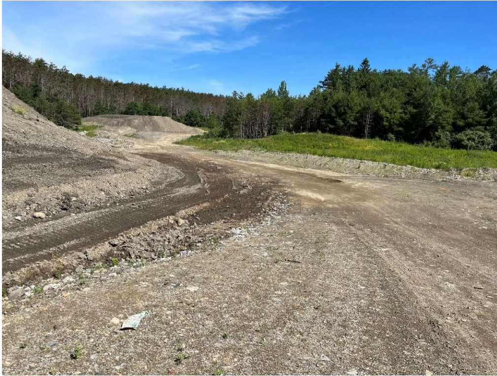
Photo 3 – Eastern slope and access road.
