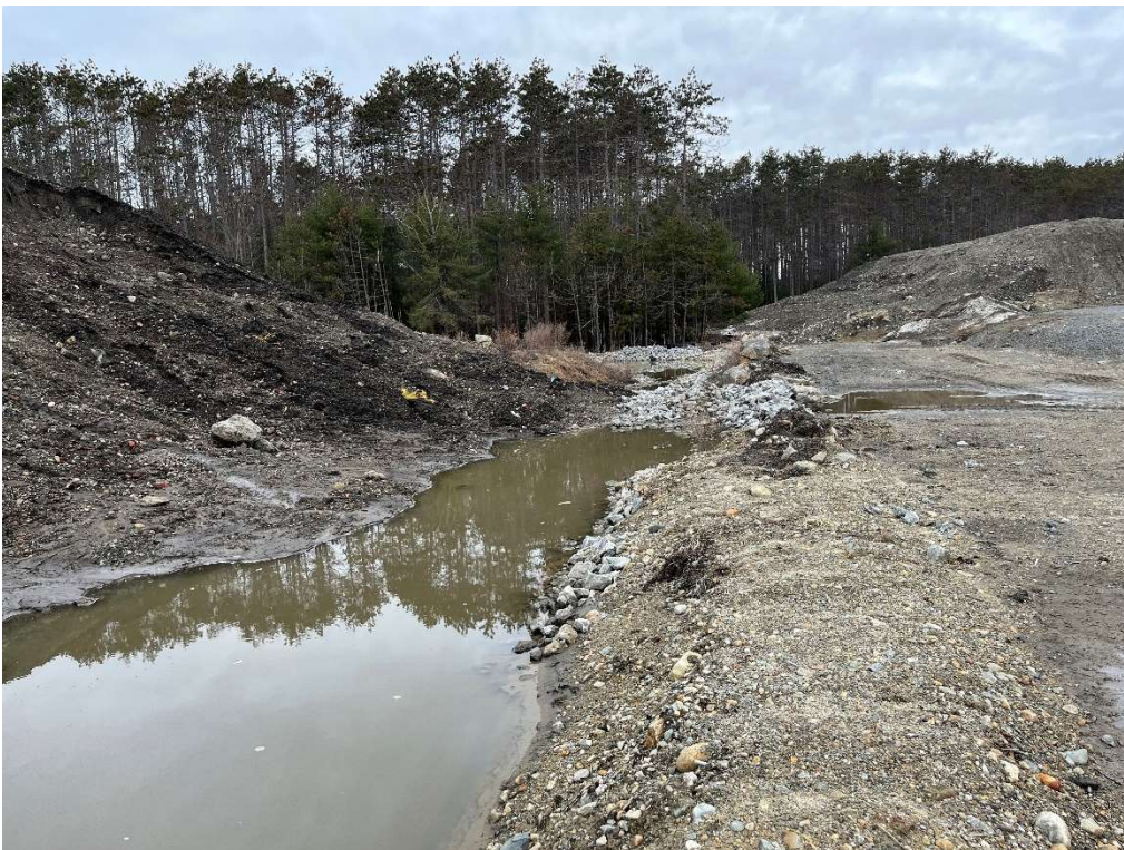
Photo 4 – Swale between temporary stormwater basin and temporary rip rap settling area.
