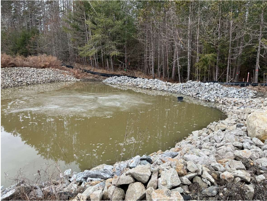
Photo 5 - Temporary rip rap settling area.
