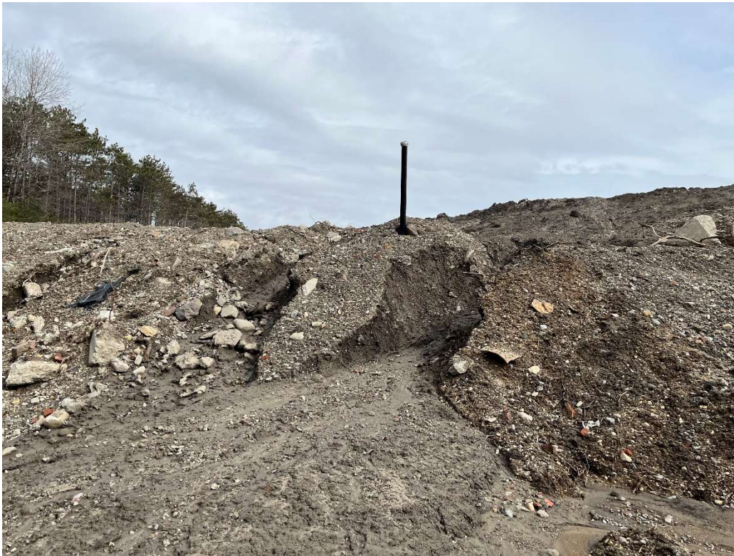
Photo 9 – Grading at monitoring well.
