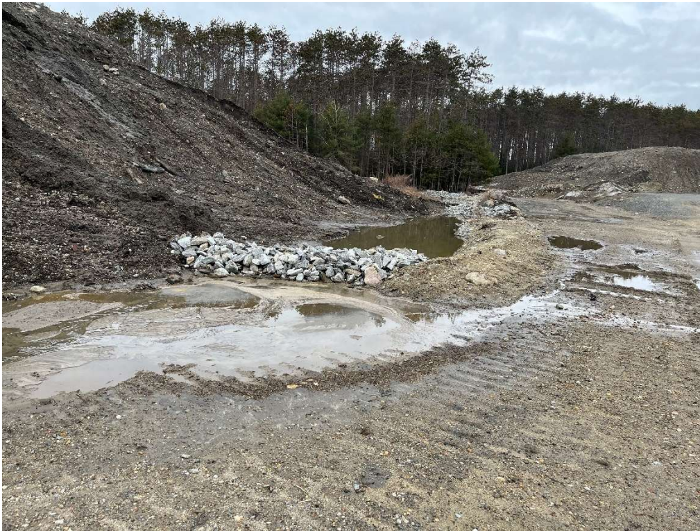
Photo 3 – Swale and check dams between temporary stormwater basin and temporary rip rap settling area.
