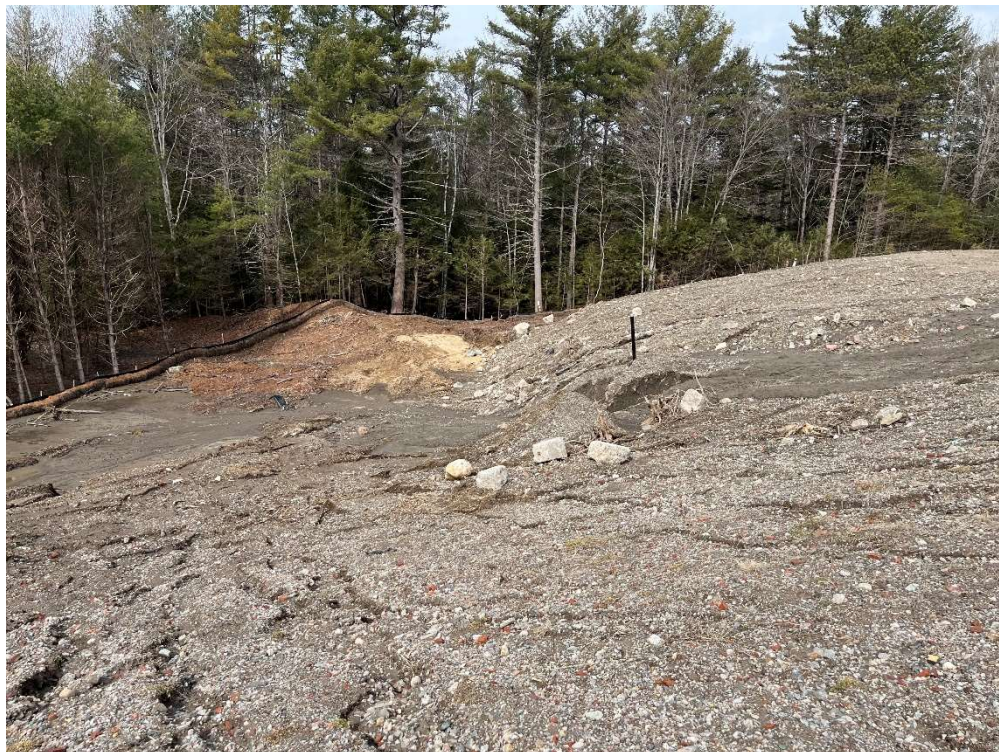
Photo 8 – Southwestern slope and erosion control.
