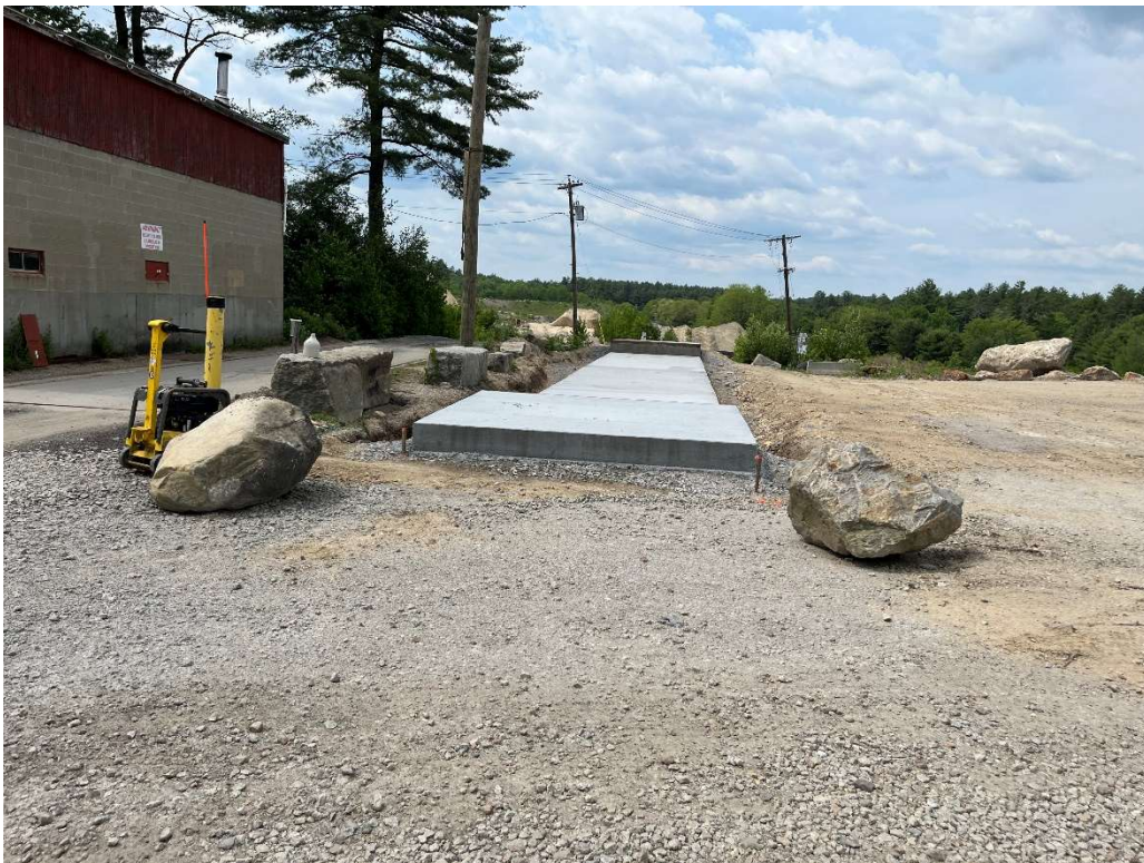
Photo 14 – Concrete pad for new scale.
