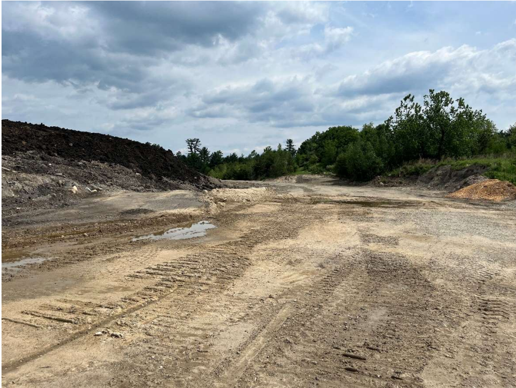
Photo 1 – Eastern slope and access road.
