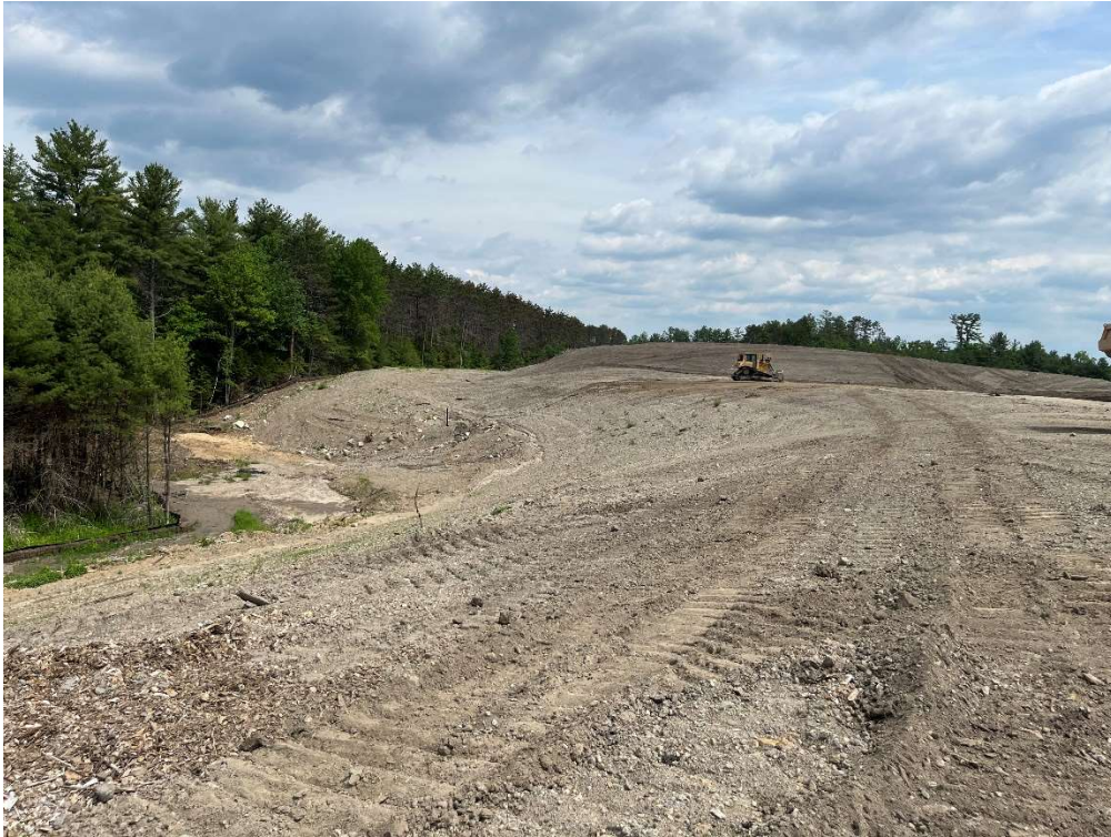
Photo 10 – Southwestern slope and erosion control.
