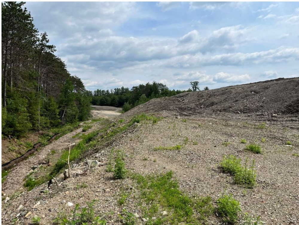
Photo 9 – Slope and erosion control at western limits of the Site.
