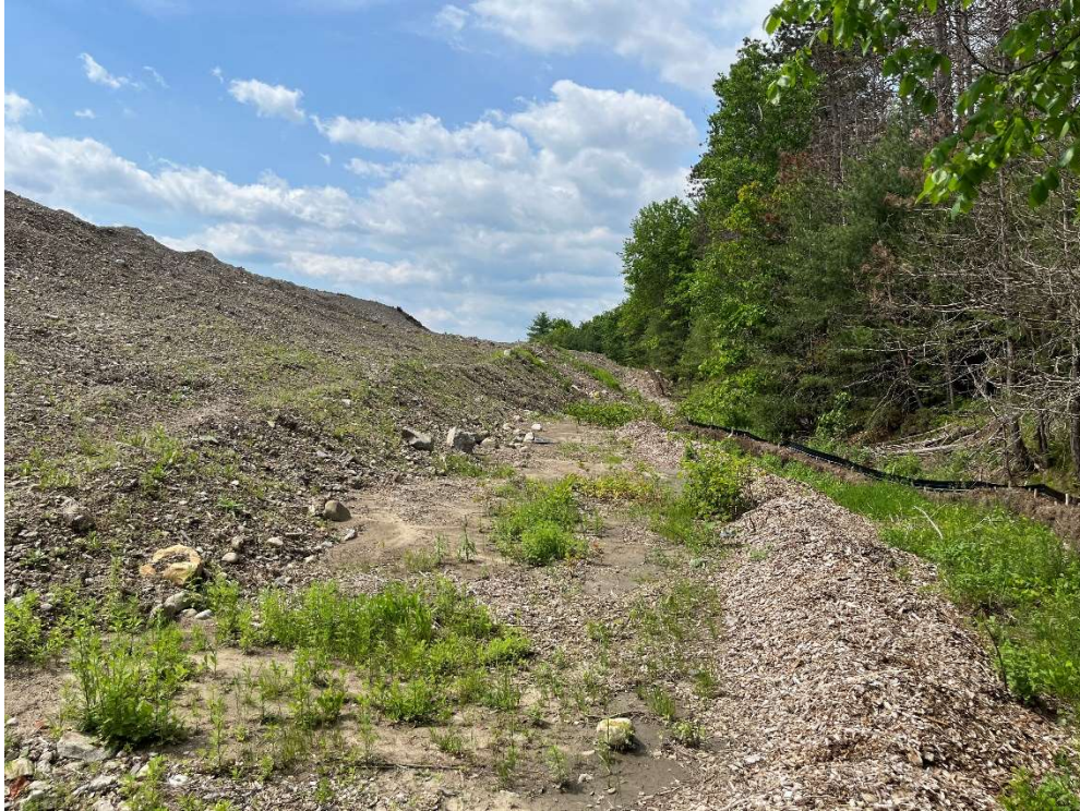
Photo 8 – Representative view of erosion control on the western limits of the Site.
