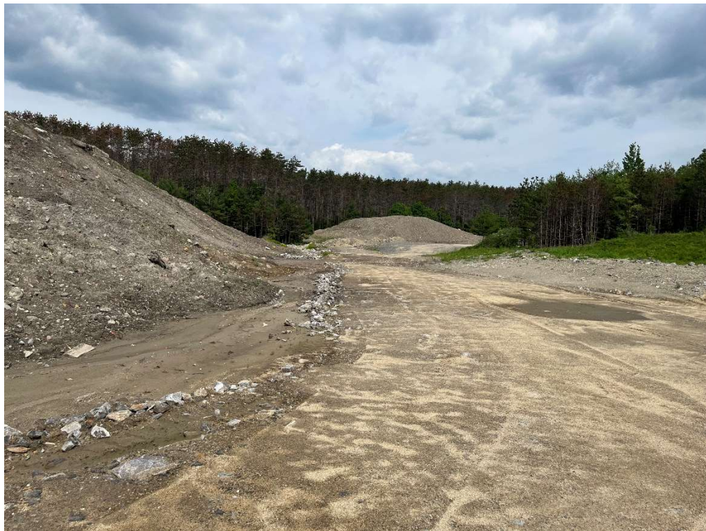
Photo 3 – Eastern slope and completed access road.
