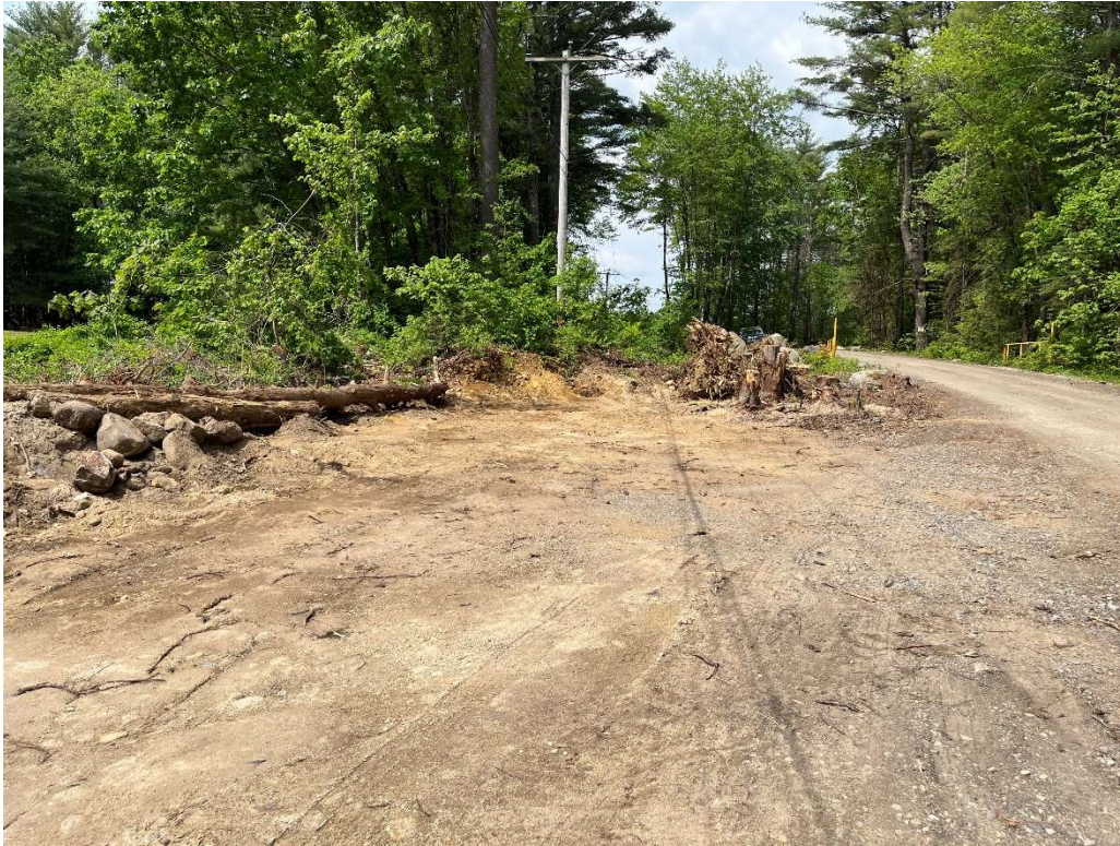
Photo 15 – Clearing and tree removal at access road.
