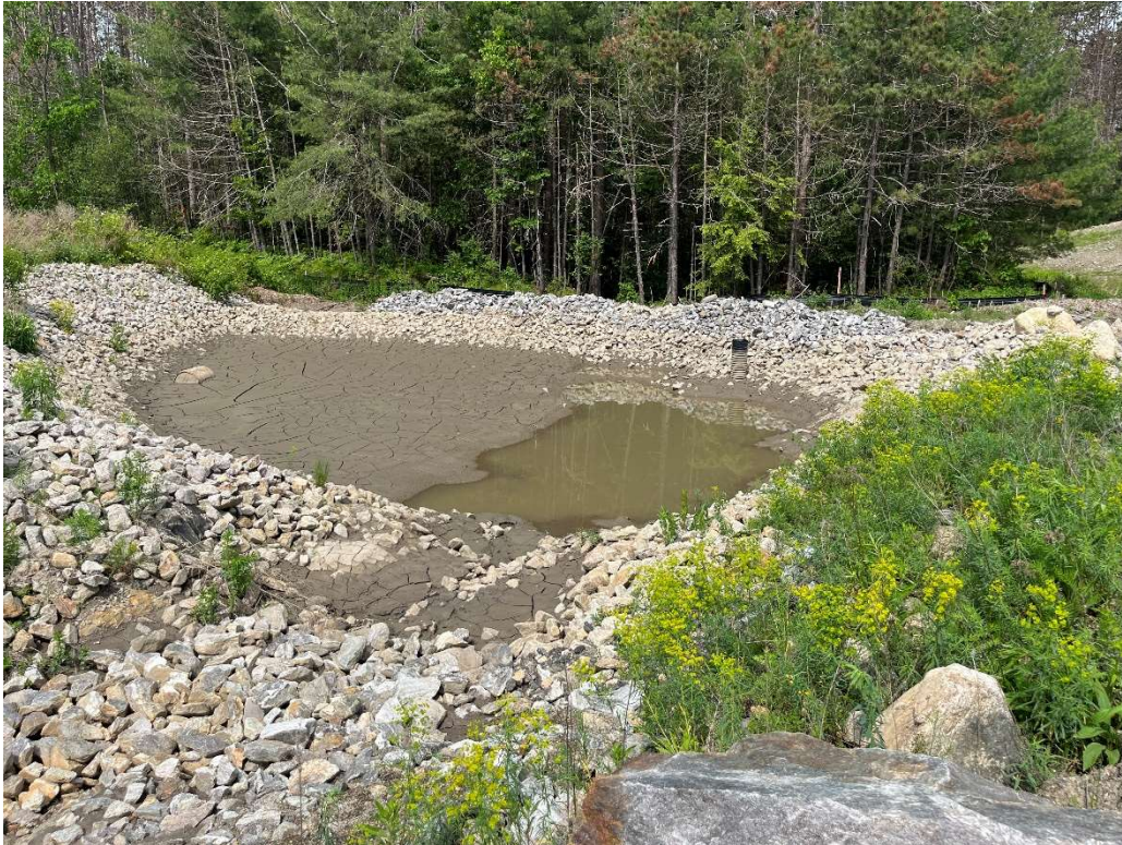
Photo 7 - Temporary rip rap settling area.
