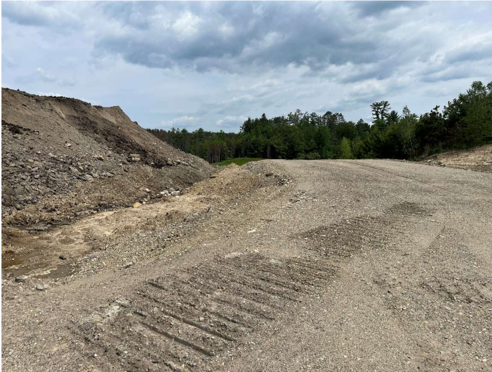
Photo 2 – Eastern slope and completed access road.
