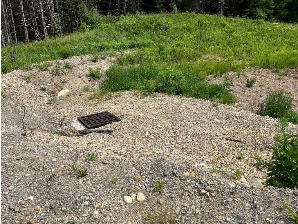
Photo 4 – Temporary stormwater overflow catch basin.
