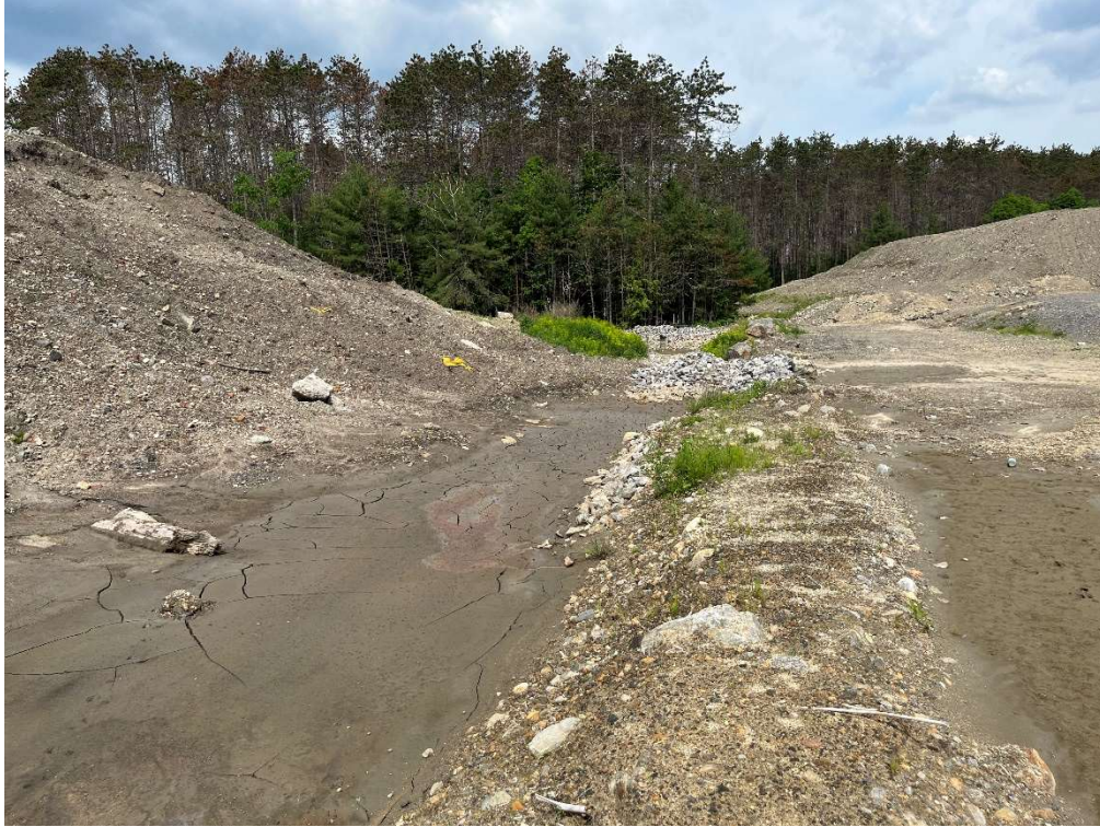
Photo 5 – Swale and check dams between temporary stormwater basin and temporary rip rap settling area.
