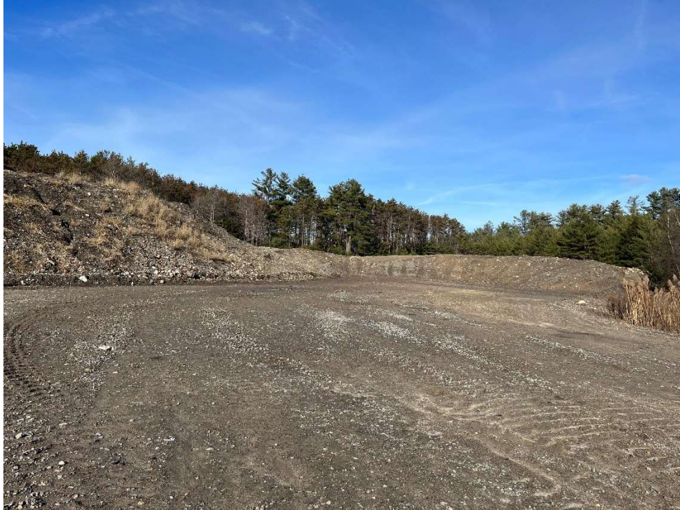
Photo 10 - Material placed and graded at the northern limits of the site.
