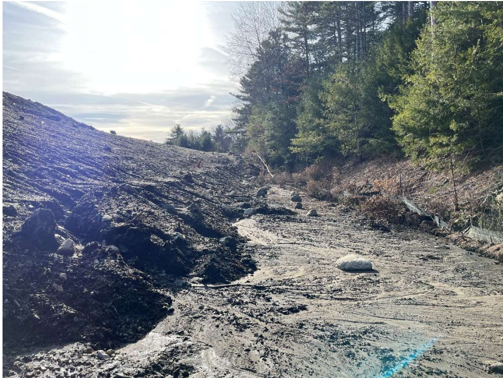
Photo 11 –Erosion control with sediment buildup on the western limits of the Site.
