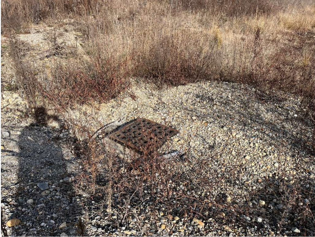
Photo 7 – Temporary stormwater overflow catch basin.
