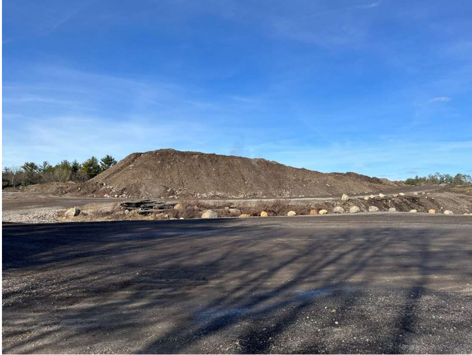
Photo 3 –Material placed and graded at the center of the Site with grading for truck access
