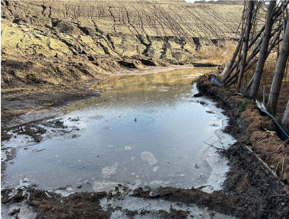
Photo 5 – Standing water at the base of the southwestern slope.
