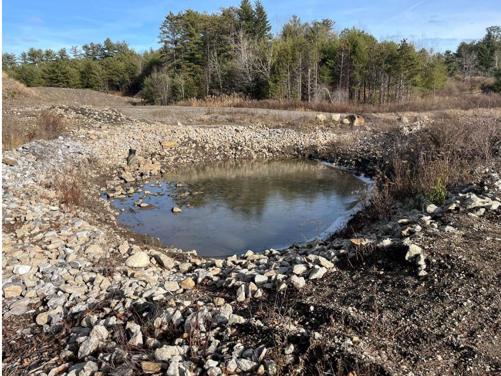
Photo 9 - Temporary rip rap settling area.
