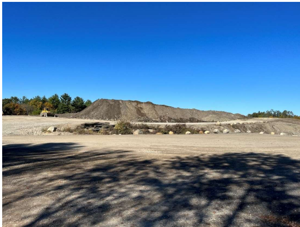
Photo 12 –Material placed and graded at the center of the Site with grading for truck access
