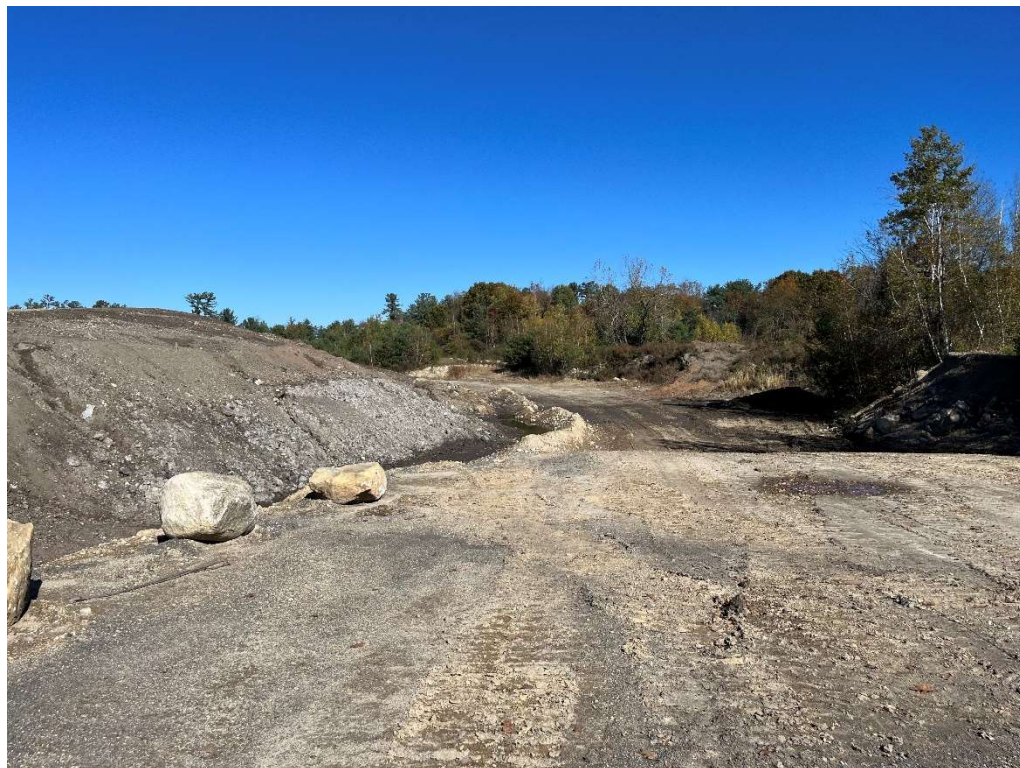
Photo 2 – Temporary swale and access road.
