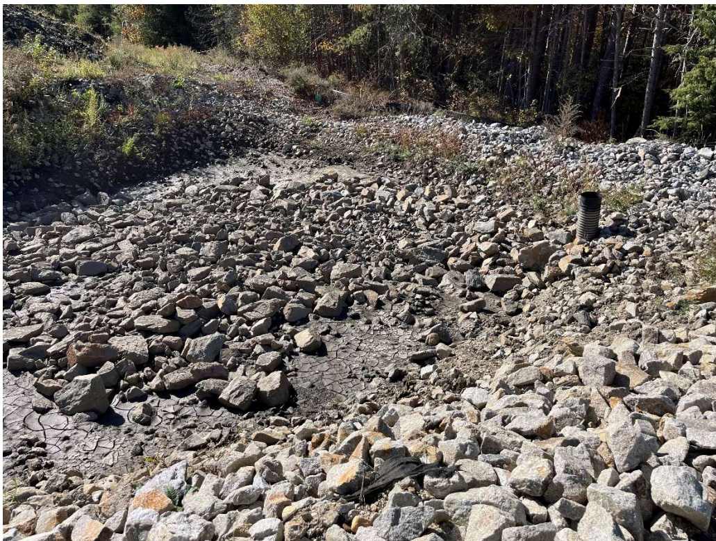
Photo 8 - Temporary rip rap settling area.
