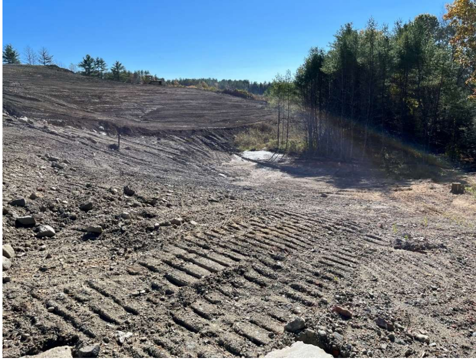
Photo 11 – Grading at monitoring well and erosion control cleared of sediment at southwestern limits of the Site.
