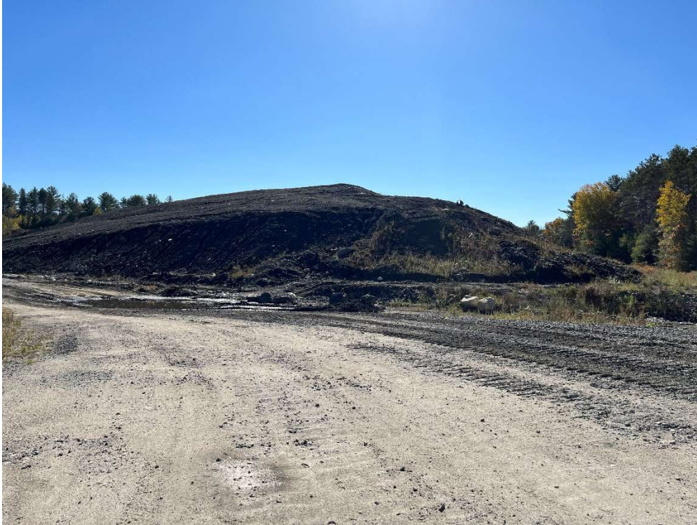
Photo 3 – Northern slope with rill erosion.
