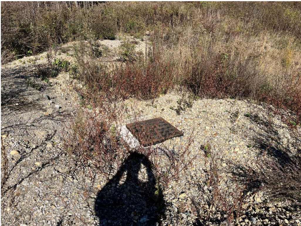
Photo 4 – Temporary stormwater overflow catch basin.
