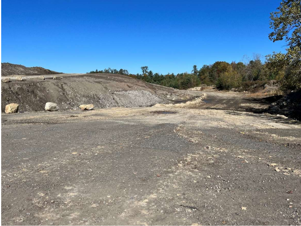
Photo 1 – Eastern slope and access road.
