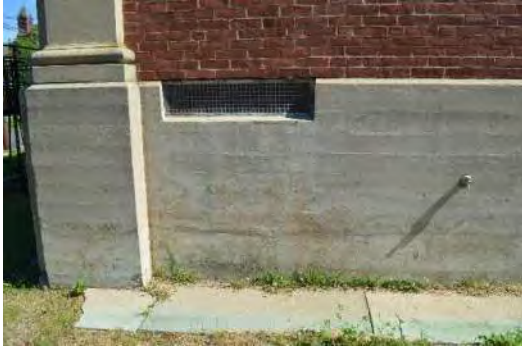
Northwest Corner (facing Murdock Avenue)
