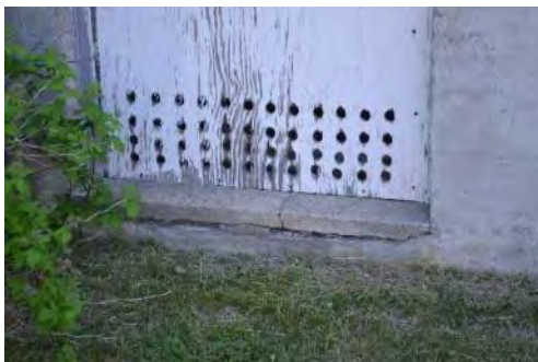
Concrete Windowsill (Basement)
