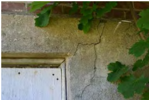
Concrete Wall at Window (Basement)
