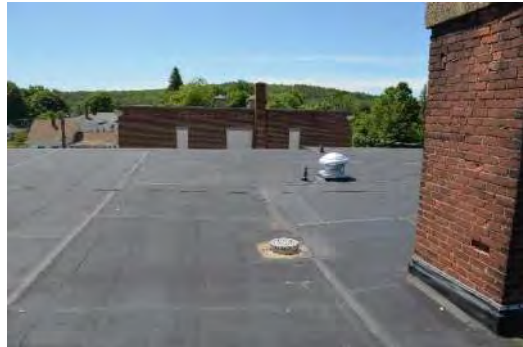
Existing Roof, Chimney and Roof Drain (Southeast Corner)
