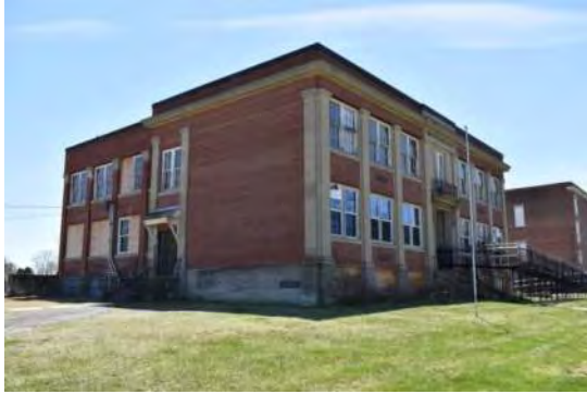
Northwest Corner (facing Murdock Avenue)
