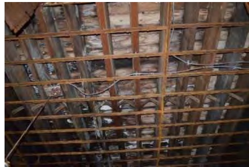
Second Floor Framing (without tin ceiling)
