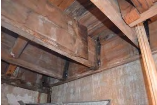
Existing Roof Framing (Attic Space)
