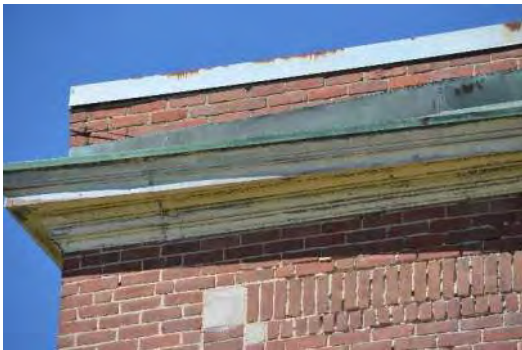
Metal Clad Cornice (Southeast Corner)
