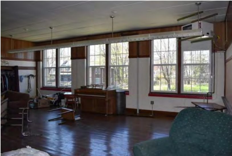
First floor classroom space
