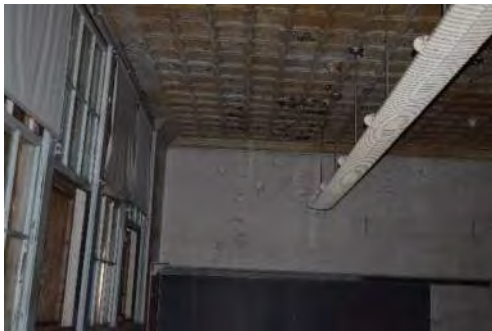
Second Floor Framing (with tin ceiling intact)
