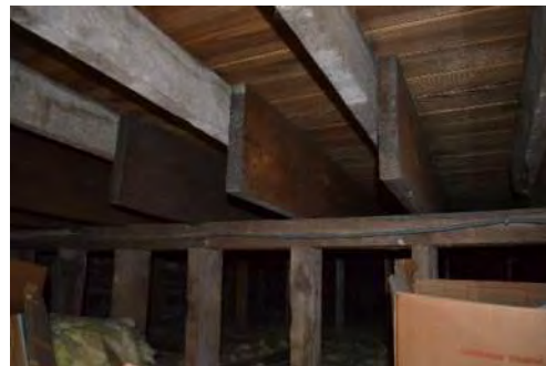
Roof Framing (within attic space)
