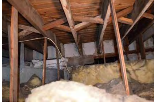
Existing Roof Framing (Attic Space)
