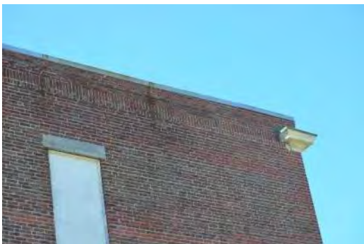
Parapet Wall (South Elevation)
