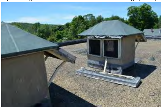
Close up of Roof Penthouse Structures (looking towards Murdock Avenue)
