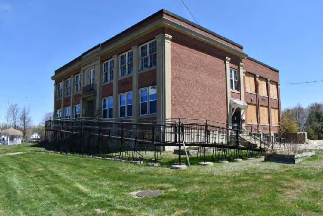
Photo 5. View northeast of the west (façade) and south elevation of Streeter School (2020).
