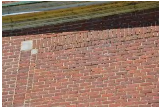
East Elevation (Top Portion of Decorative Brick Panel)
