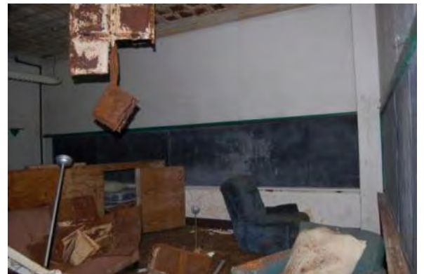
First floor classroom, west side
