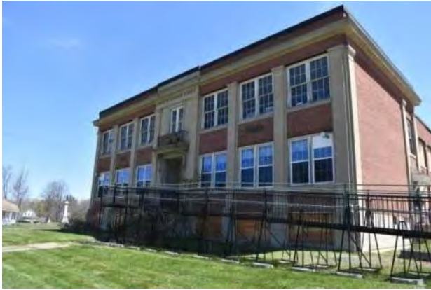
Murdoch Ave. view from southwest
