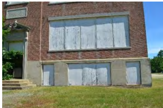
Southeast Elevation (Basement & 1 st Floor)
