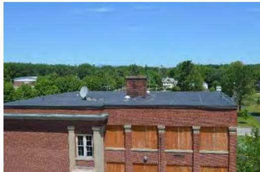
Existing Roof (Elevation)
