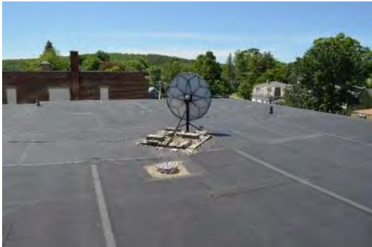
Existing Roof and Roof Drain (Southwest Corner)
