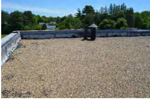
Northeast Corner of Roof
