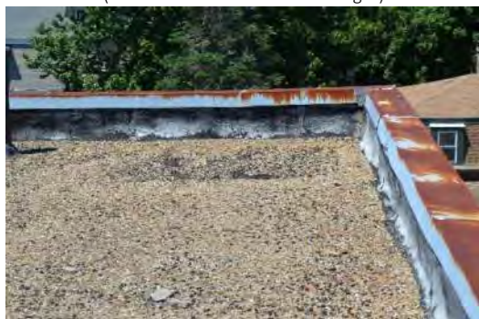
Southeast Corner of Roof (looking towards Murdock Avenue)
