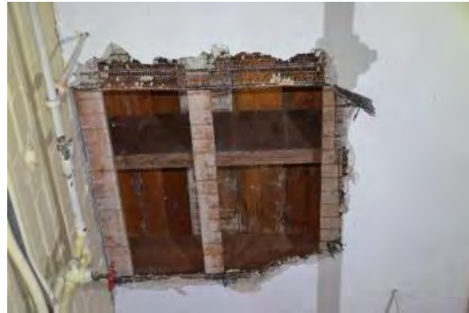
Observation Hole (Exist. 1 st Floor Framing)
