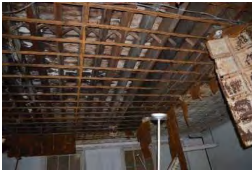
Second Floor Framing (without tin ceiling)
