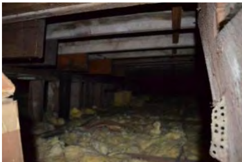
Roof Framing (within attic space)
