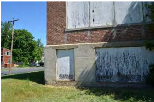
Southwest Elevation (Basement & 1 st Floor)
