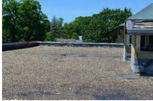
Southwest Corner of Roof (Wood Framed Penthouse on Right)
