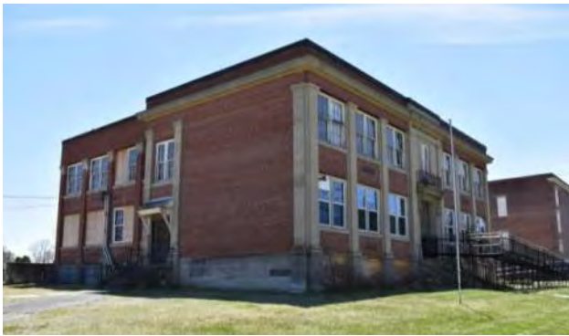
North elevation from west
