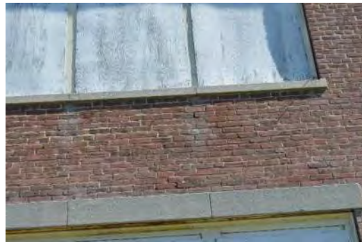
South Elevation (Brick Panel between 1 st and 2 nd Floors)
