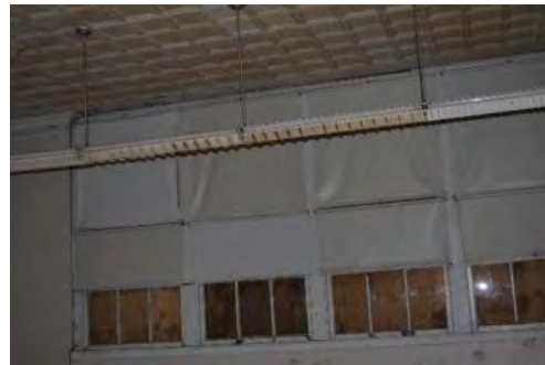
Second Floor (facing the Exterior Wall)
