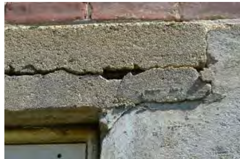
Concrete Lintel at Window (Basement)
