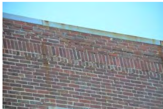
Parapet Wall (South Elevation)
