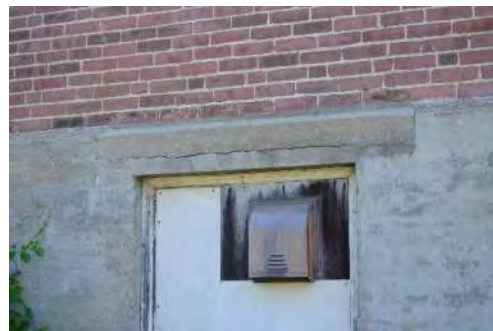
Concrete Lintel at Window Infill (Basement)
