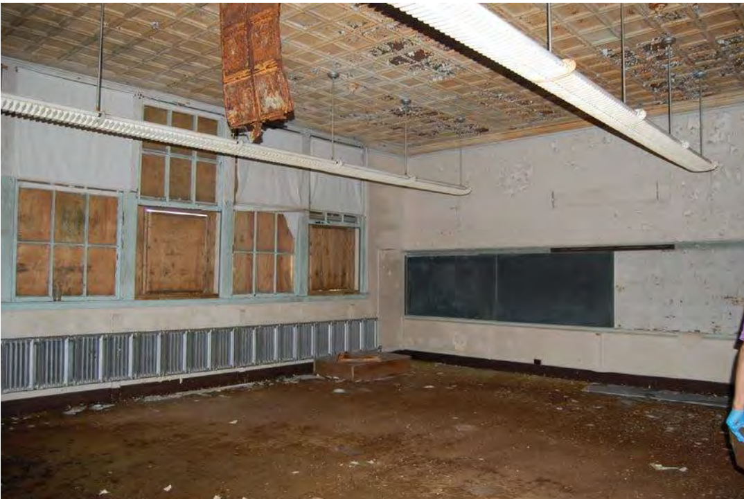
Photo 3. View southwest of the southwest classroom, second floor of Poland School (2020).
