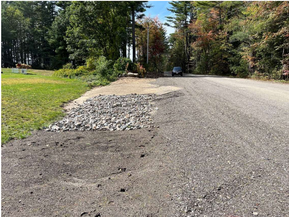
Photo 14 – Rip rap placed at the access road entrance.
