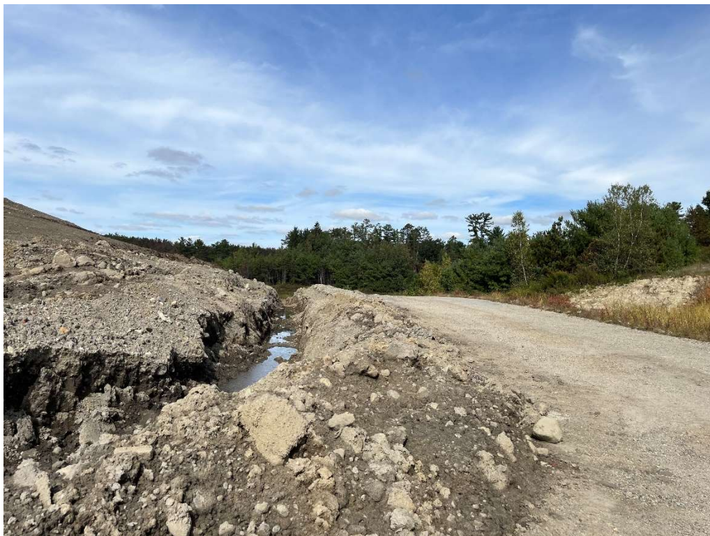
Photo 2 – Temporary swale and access road.
