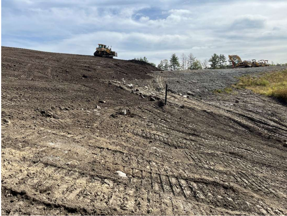
Photo 13 – Grading at monitoring well.
