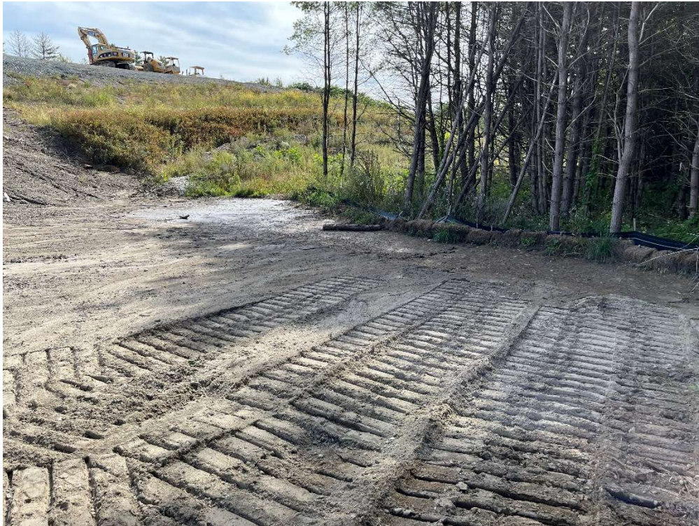
Photo 11 –Erosion control cleared of sediment at southwestern limits of the Site.
