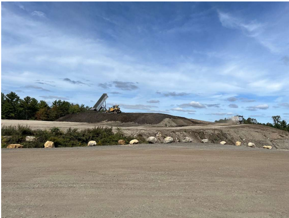
Photo 12 –Material being placed and graded at the center of the Site.
