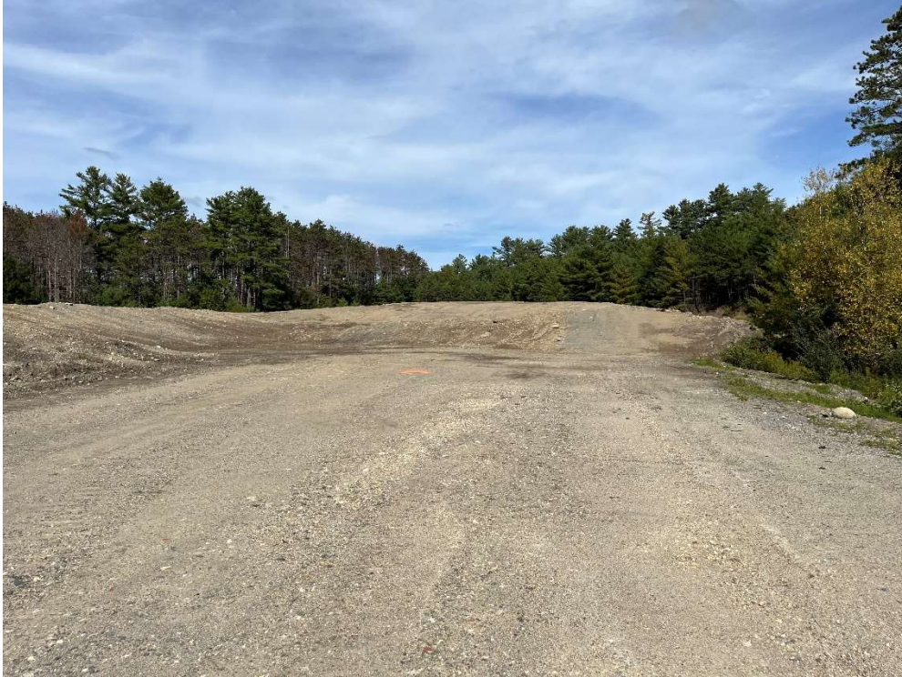
Photo 9 – Material placed and graded at the northern limits of the site.
