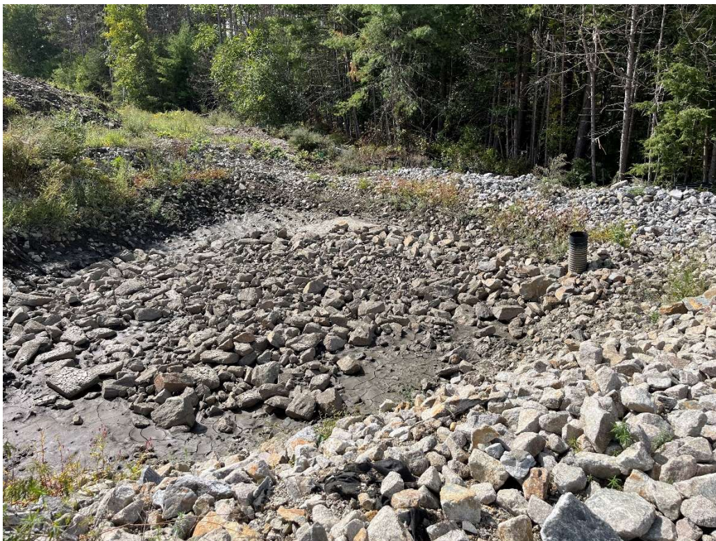
Photo 8 - Temporary rip rap settling area.
