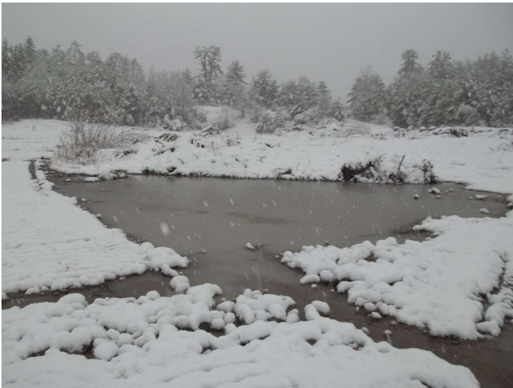
Photo 2 – Temporary Stormwater Basin. 4' high berm with rip rap overflow not yet constructed.
