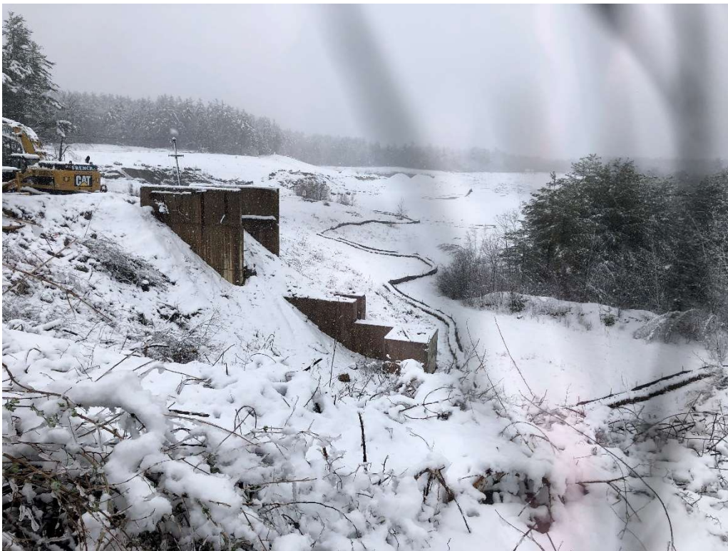
Photo 6 - Existing slope and erosion control at the southern limits of the Site.
