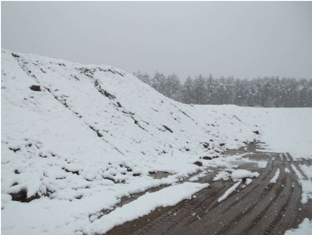
Photo 1 – Eastern slope and existing access road.
