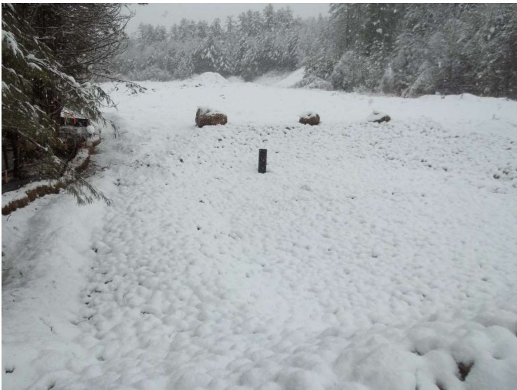
Photo 4 - Temporary rip rap settling area.
