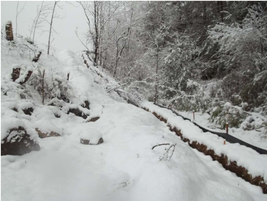
Photo 5 - Representative view of erosion control on the western limits of the Site.
