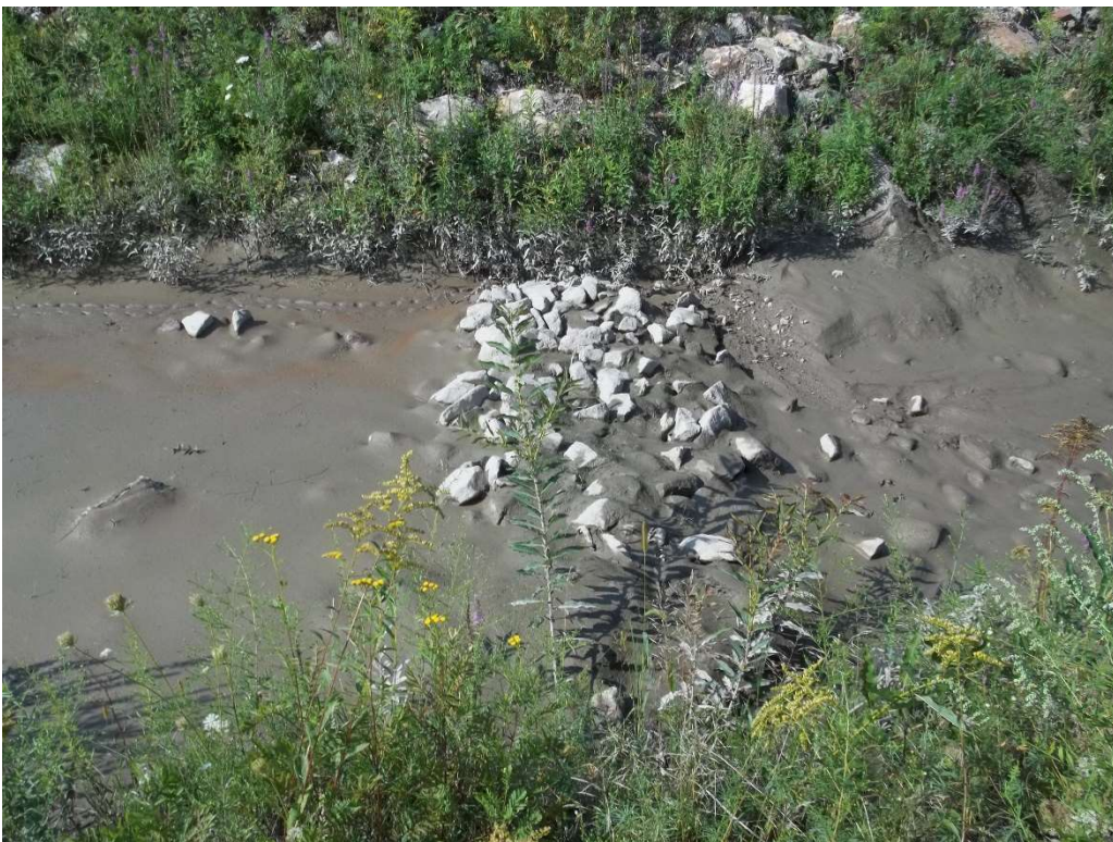
Photo 6 - Check dam and sediment buildup between temporary stormwater basin and temporary rip rap settling area.
