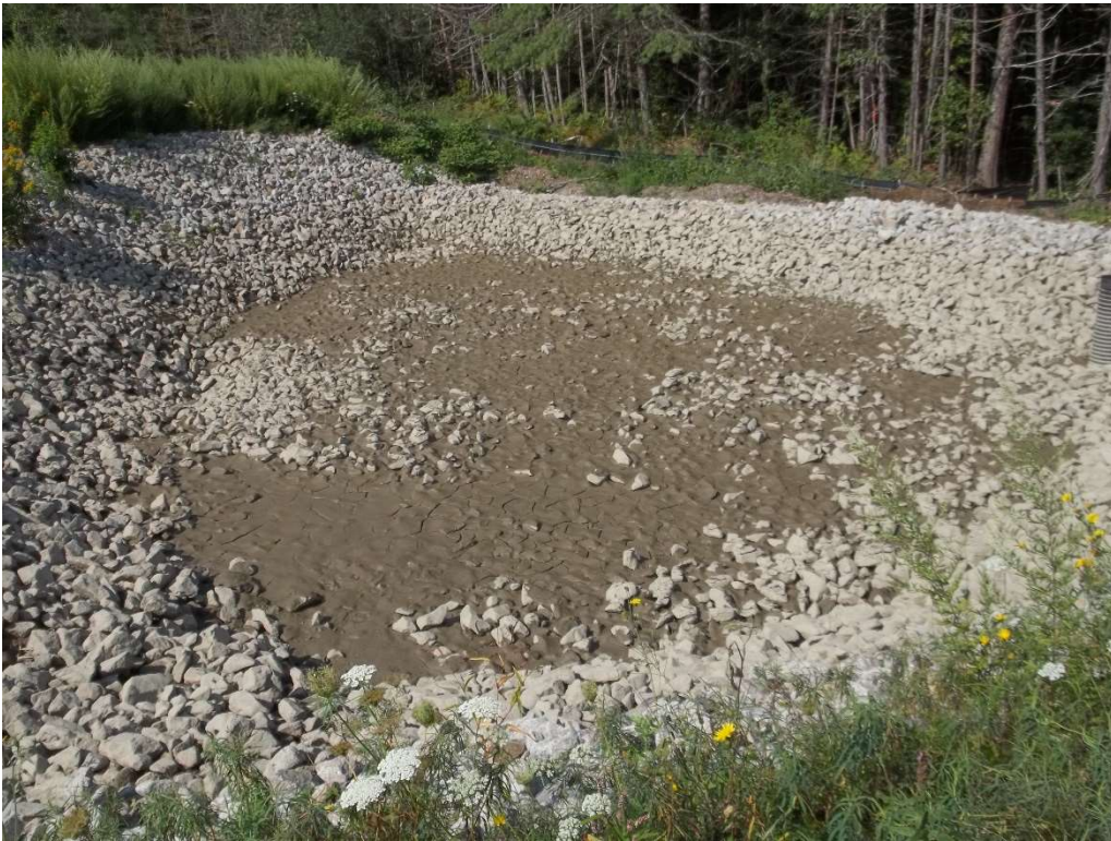
Photo 7 - Temporary rip rap settling area.
