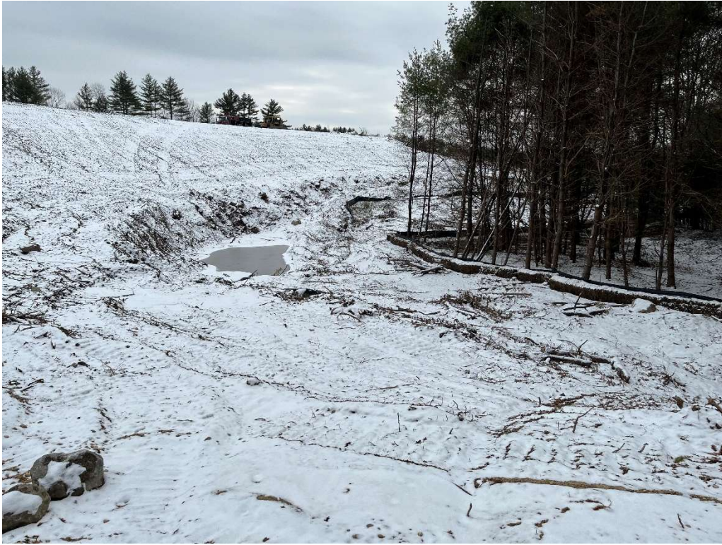
Photo 9 – Southwestern slope and erosion control.
