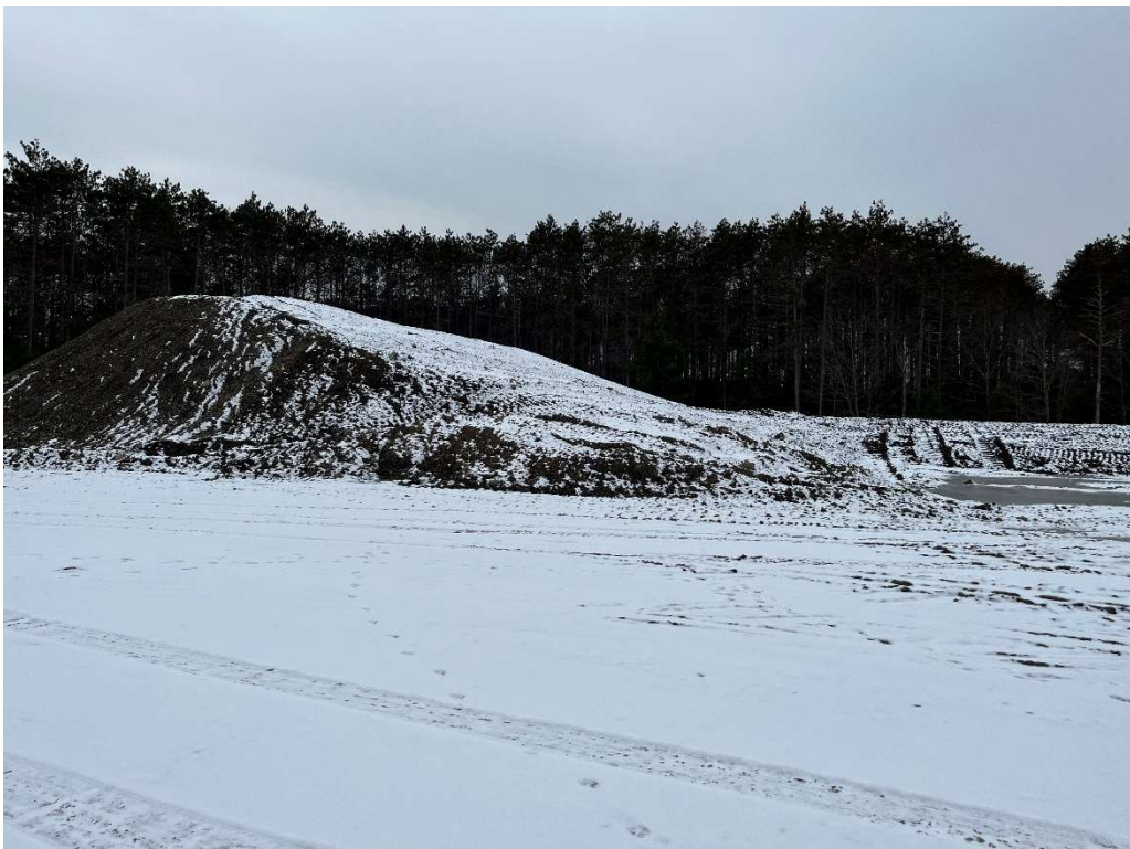
Photo 6 - Material placed and graded in the northern area of the site.
