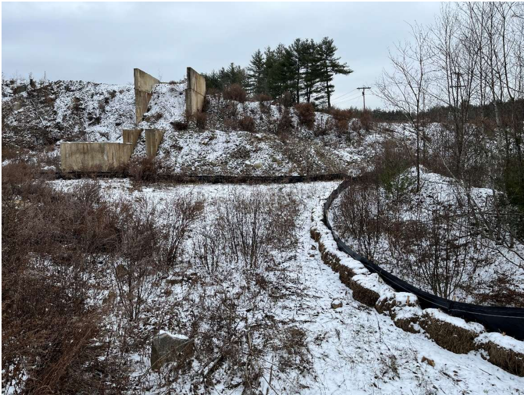
Photo 11 – Existing slope and erosion control at the southern limits of the Site.
