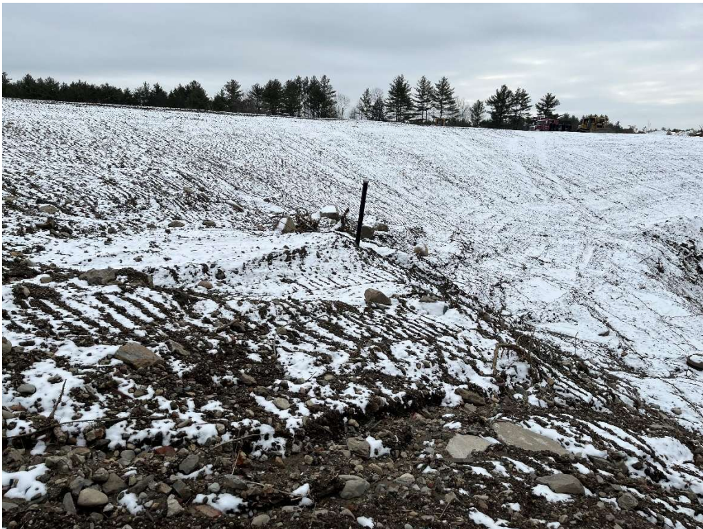
Photo 10 – Grading at monitoring well.
