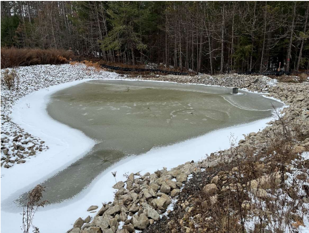
Photo 5 - Temporary rip rap settling area.
