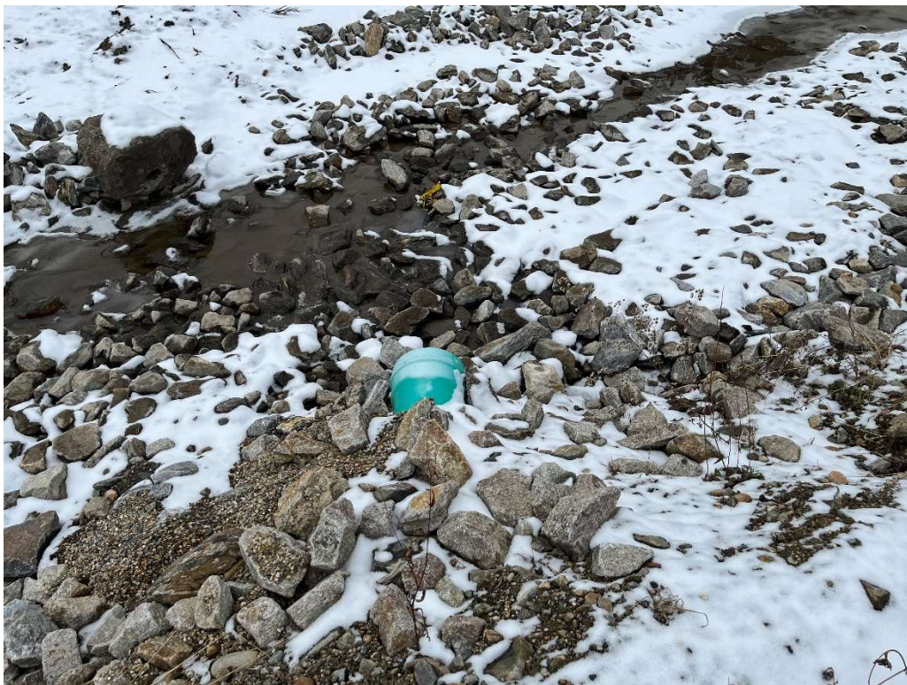
Photo 4 – Stormwater culvert under access road.
