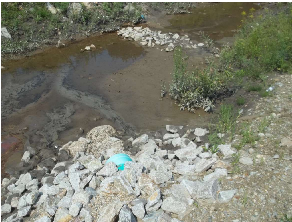
Photo 4 – Stormwater culvert under access road and sediment in swale
