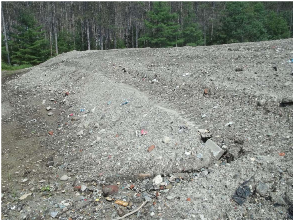
Photo 2 – Material placed and shaped on the northern section of the site.
