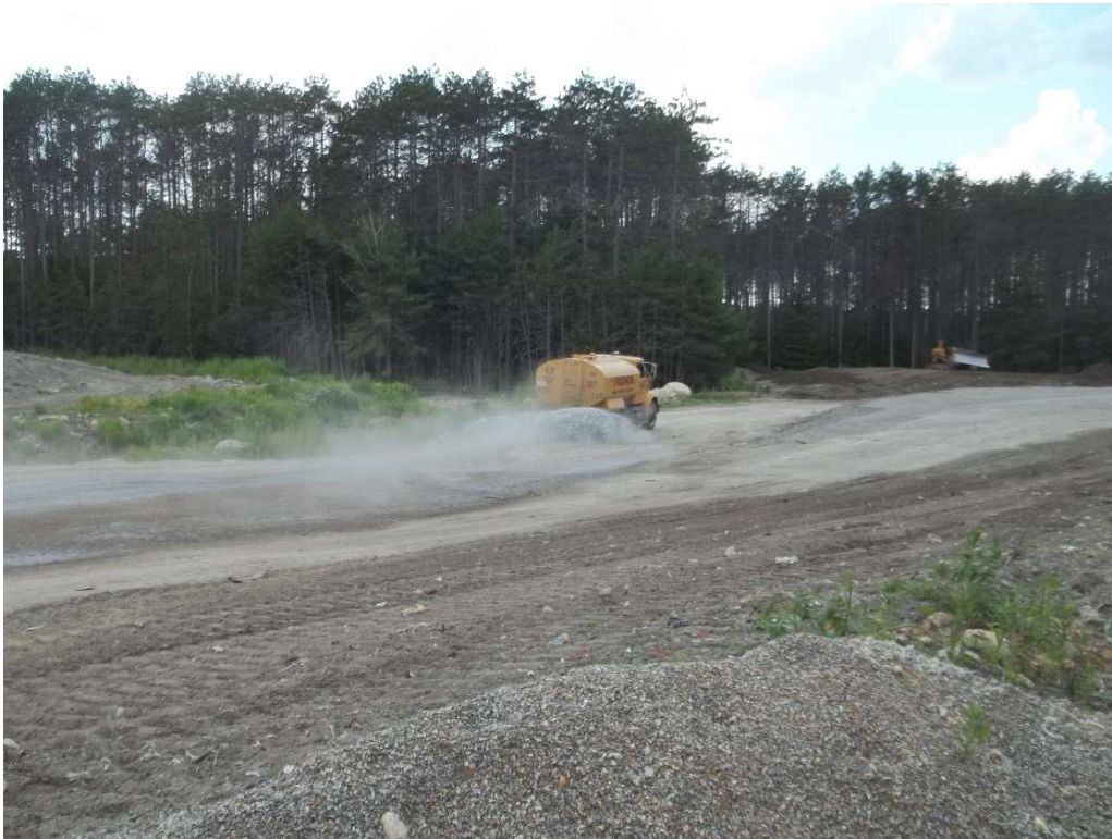
Photo 8 – Water truck dispensing water for dust control.
