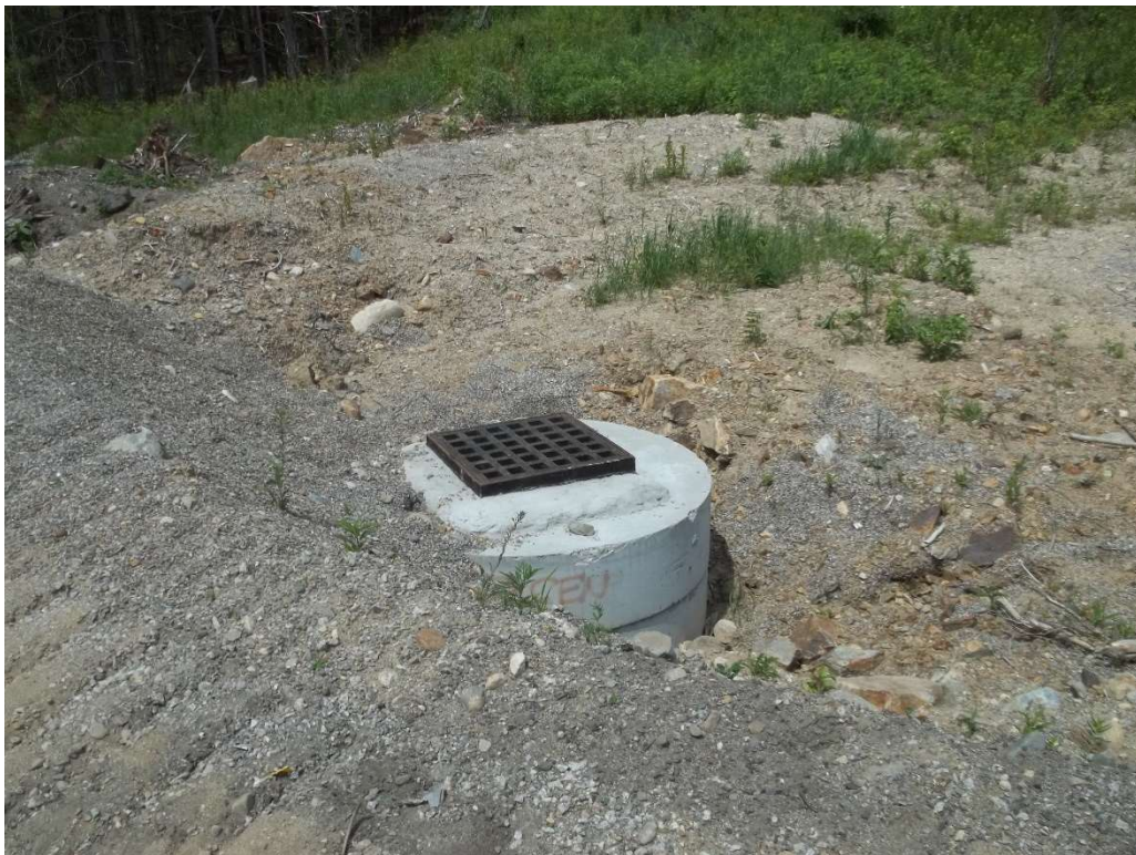
Photo 2 – Temporary Stormwater Overflow Catch Basin.
