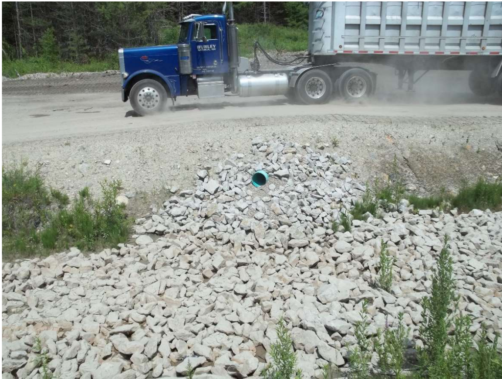
Photo 3 – Stormwater Culvert Under Access Road
