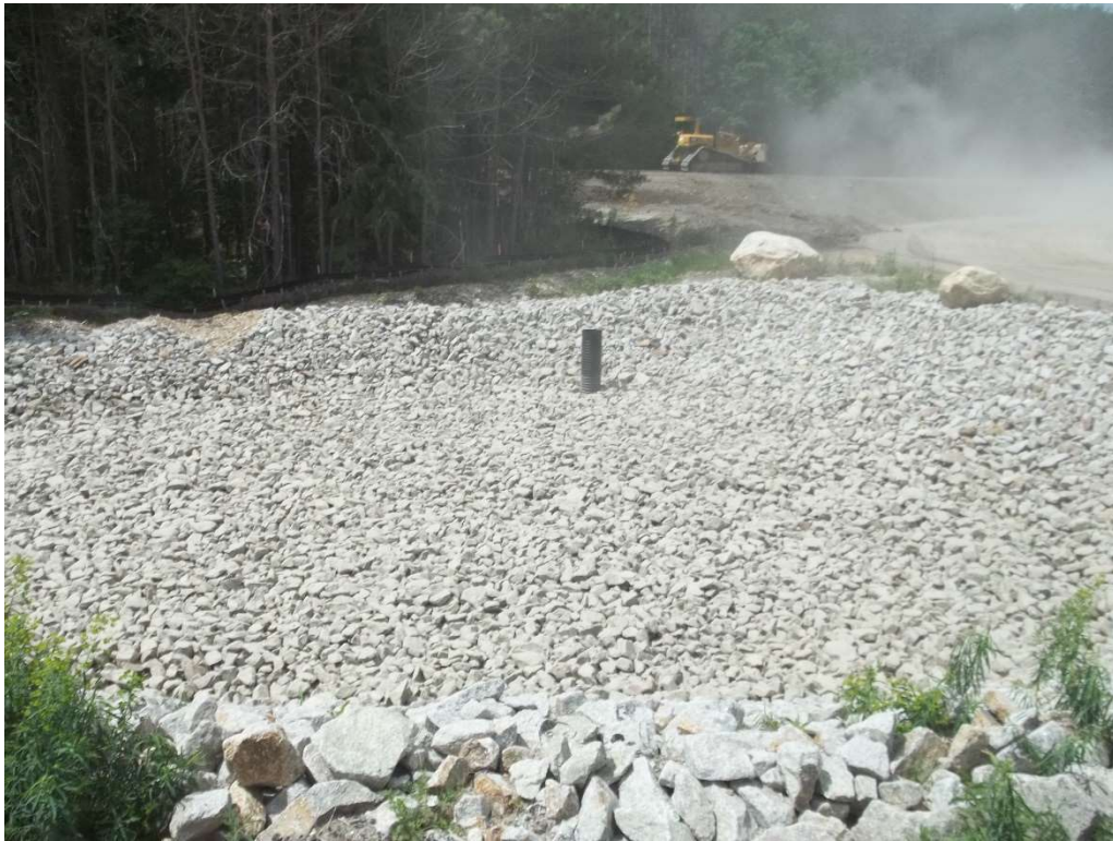
Photo 4 - Temporary rip rap settling area.
