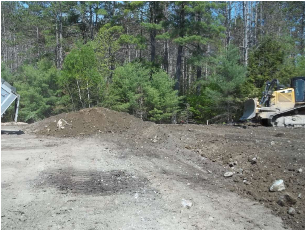
Photo 7 – Material delivered to site and placed for grading and shaping.
