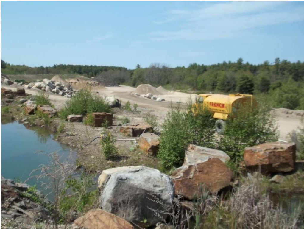
Photo 8 – Water truck collecting water from adjacent site for dust control.
