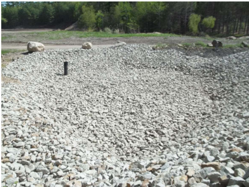
Photo 4 - Temporary rip rap settling area.
