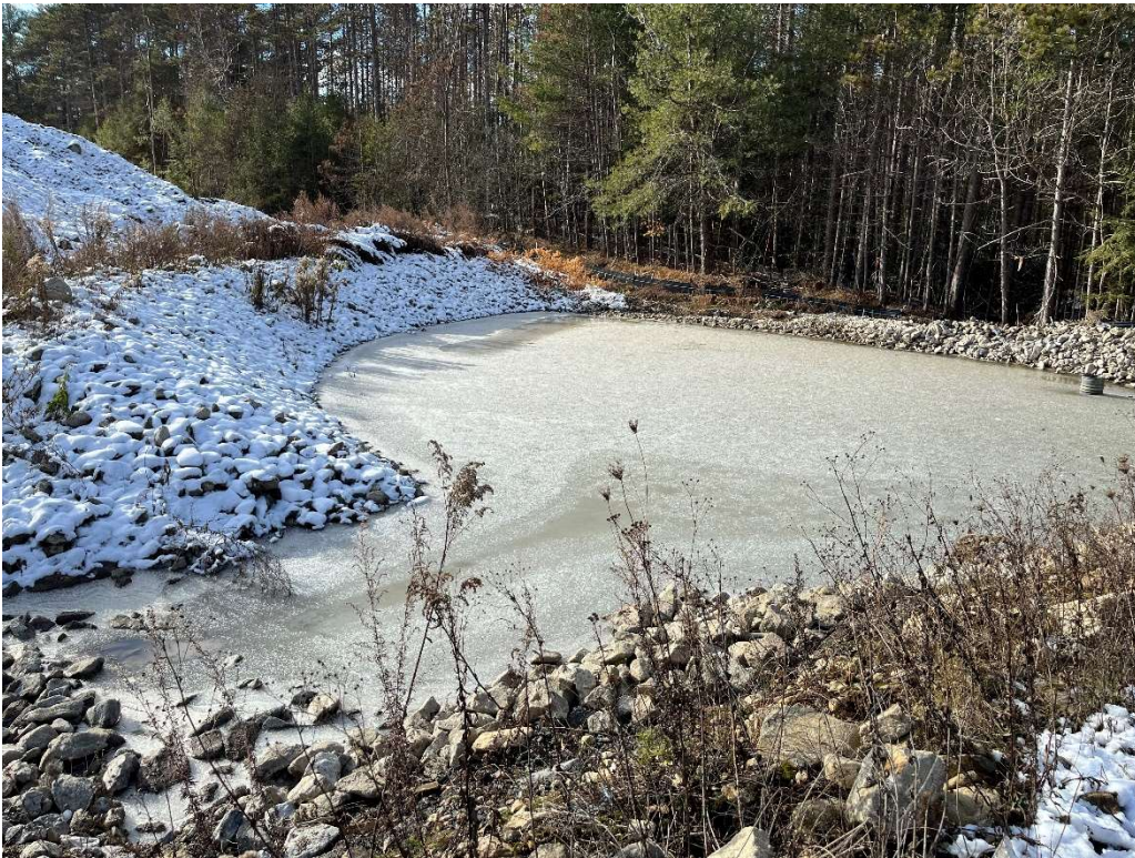
Photo 5 - Temporary rip rap settling area.
