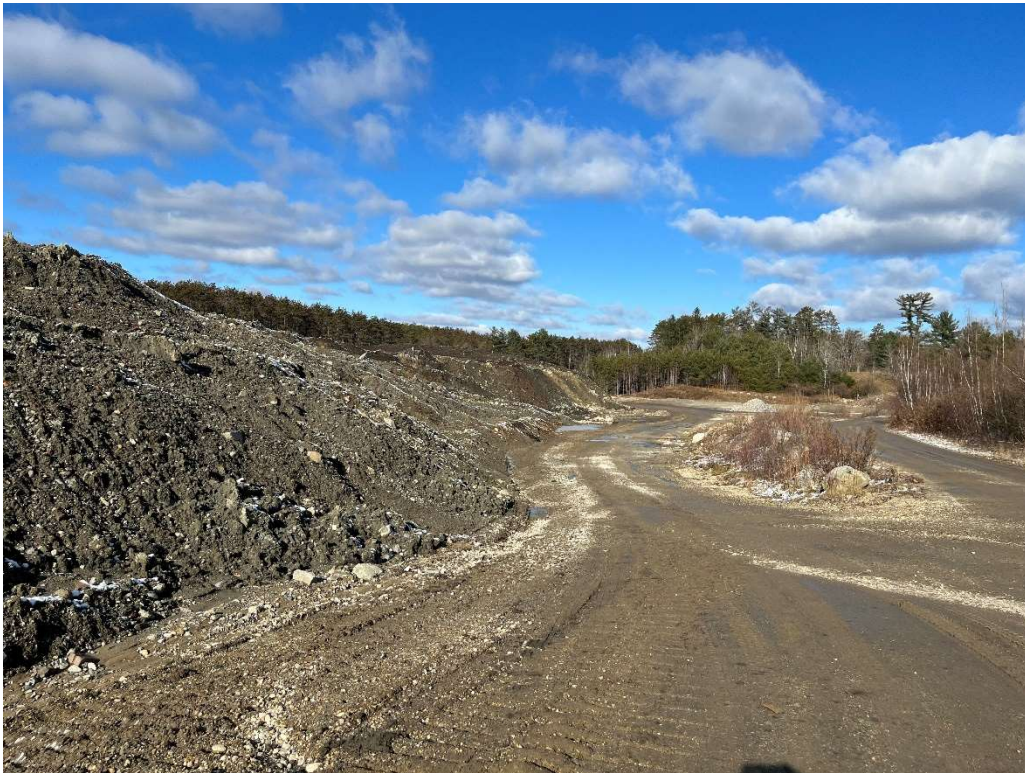
Photo 1 – Eastern slope and access road.
