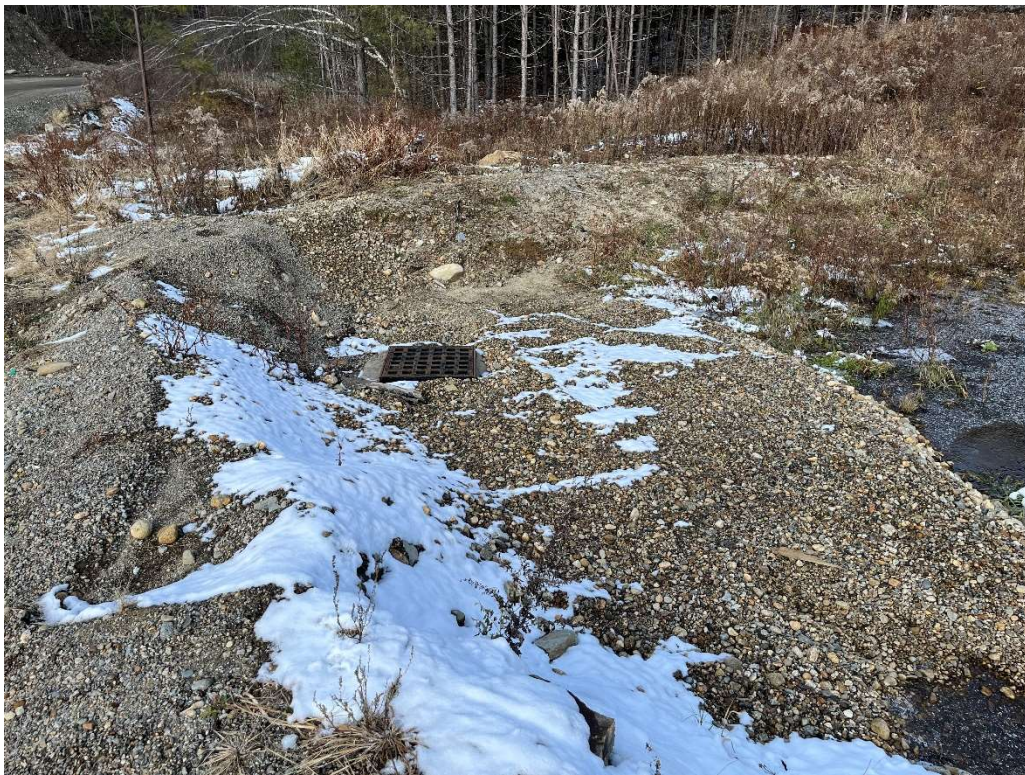
Photo 2 – Temporary stormwater overflow catch basin.
