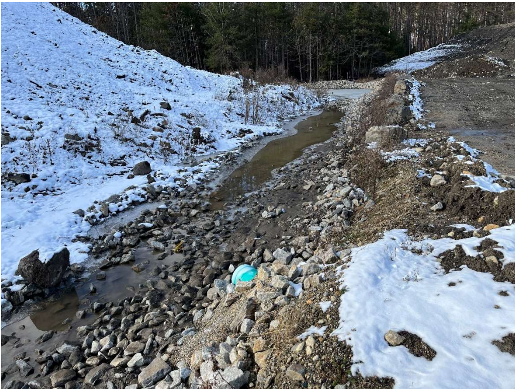
Photo 4 – Stormwater culvert under access road.
