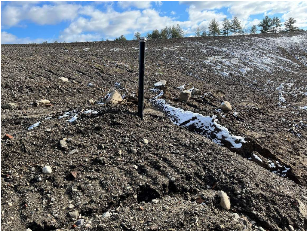
Photo 10 – Grading at monitoring well.
