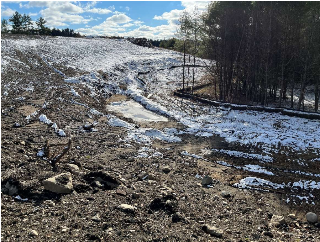
Photo 9 – Southwestern slope and erosion control.
