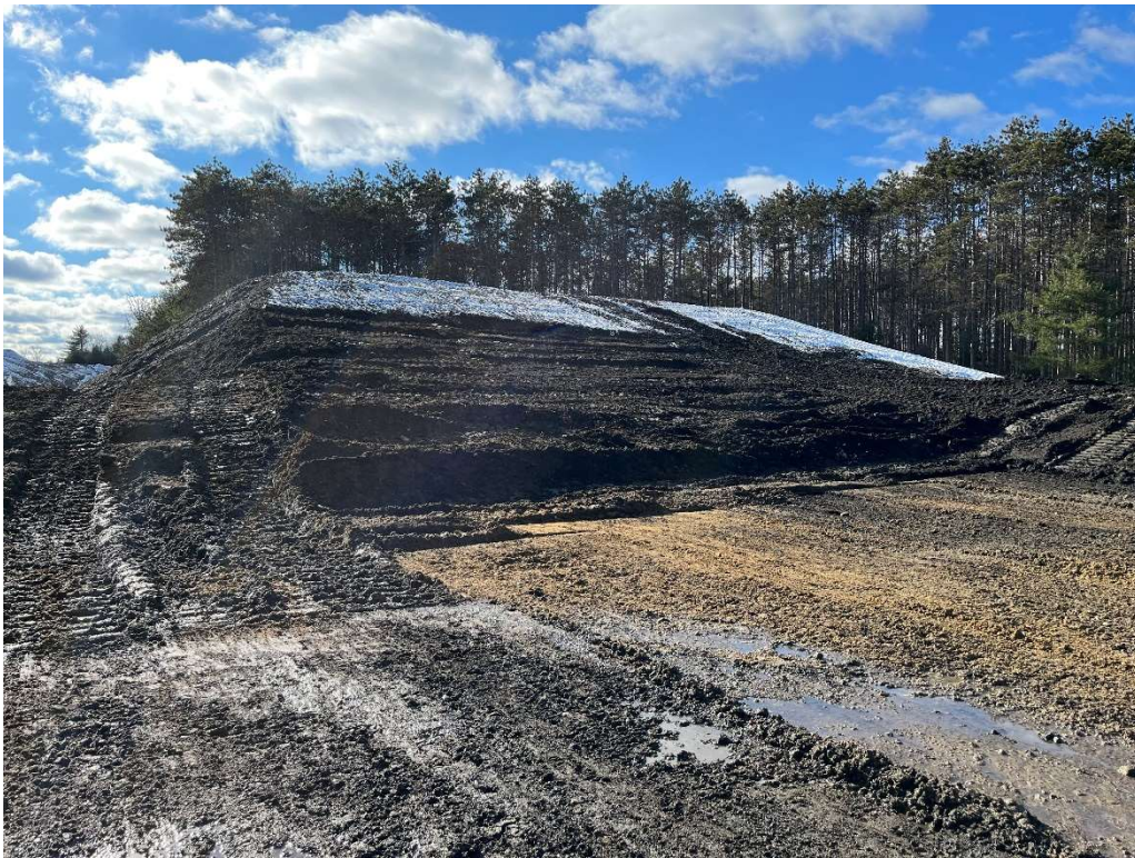
Photo 7 – Material placed and graded in the northern area of the site.
