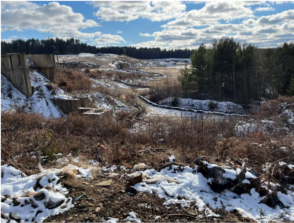
Photo 11 – Existing slope and erosion control at the southern limits of the Site.
