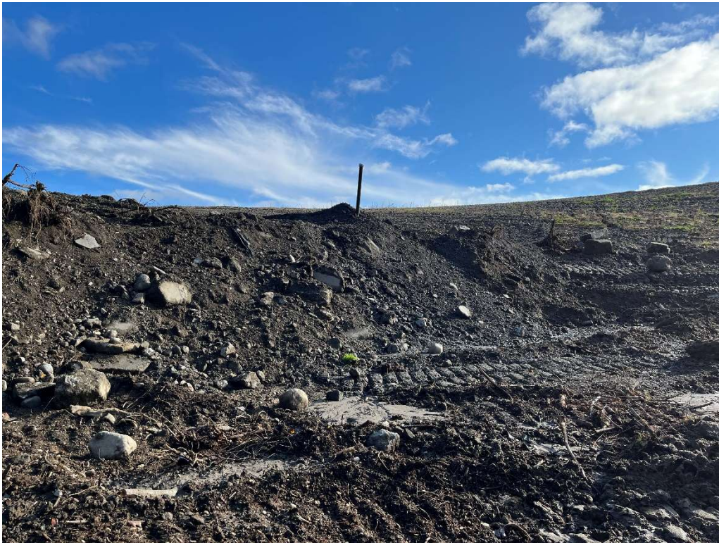
Photo 9 – Repairs and continued erosion in the subgrade slope adjacent to a monitoring well.
