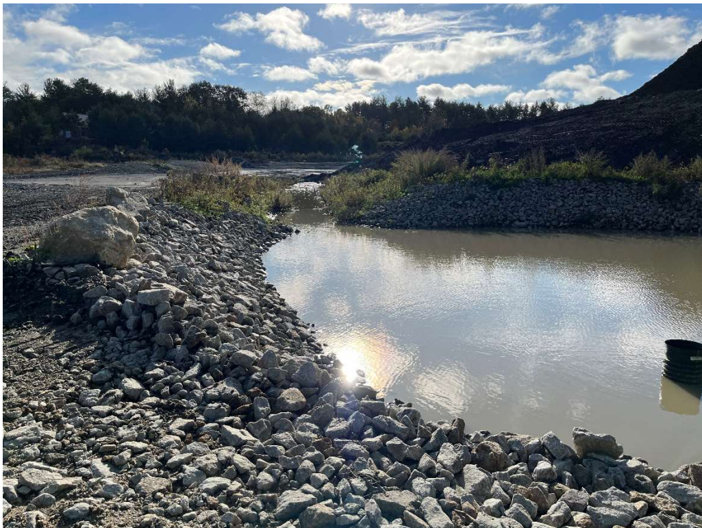
Photo 6 - Temporary rip rap settling area and swale.
