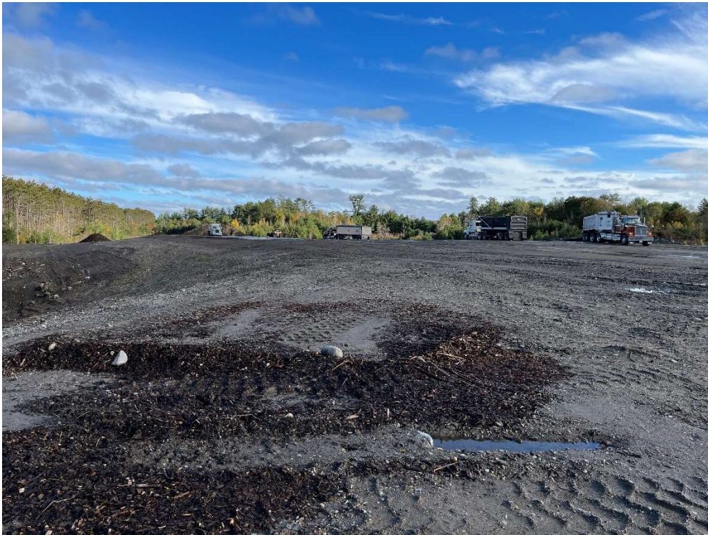
Photo 11 – Trucks queued for placing of material.
