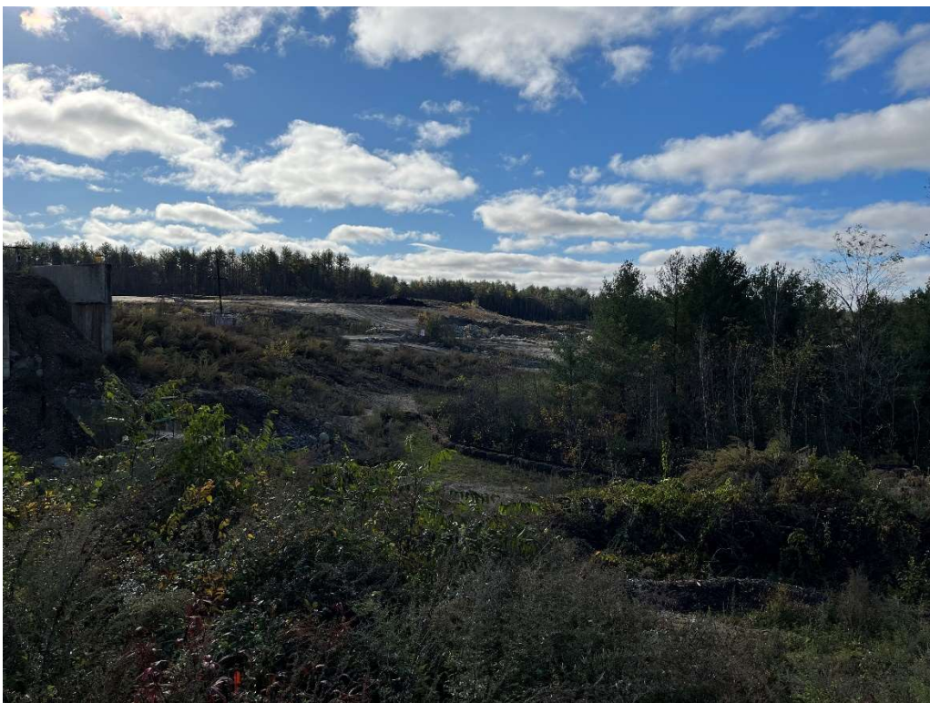
Photo 10 – Existing slope and erosion control at the southern limits of the Site.
