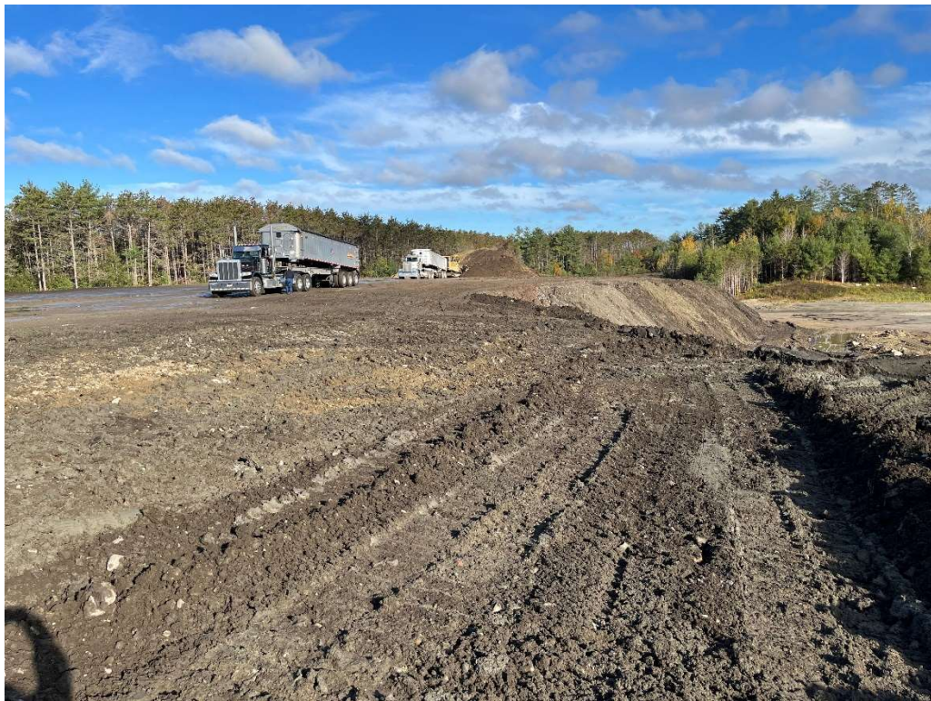
Photo 2 – Material delivered to the Site and placed for grading and shaping.
