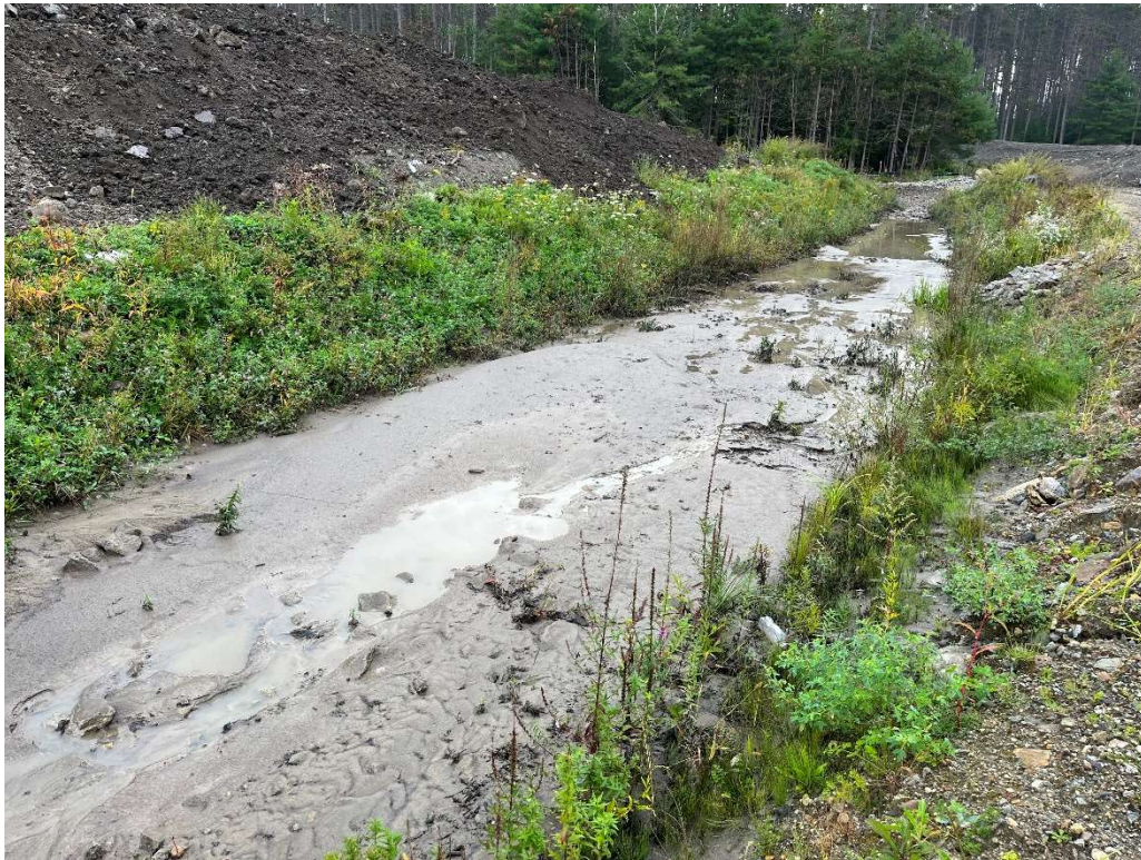
Photo 5 - Swale between temporary stormwater basin and temporary rip rap settling area.
