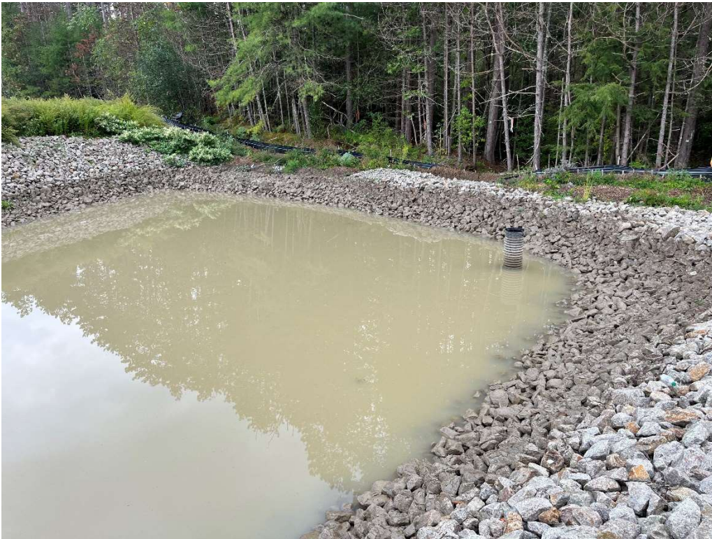
Photo 7 - Temporary rip rap settling area.
