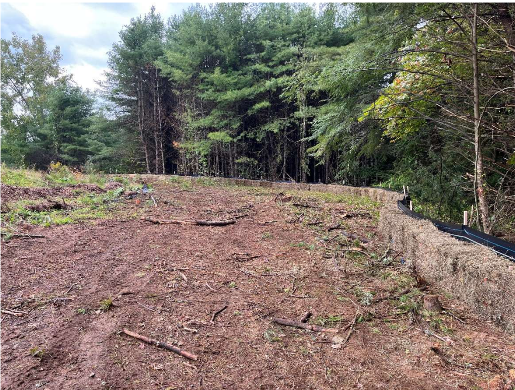
Photo 8 - Repaired erosion control at the western limits of the Site.
