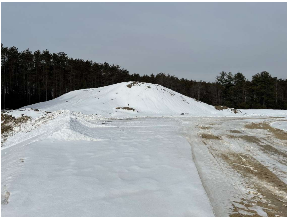
Photo 6 - Material placed and graded in the central area of the site.
