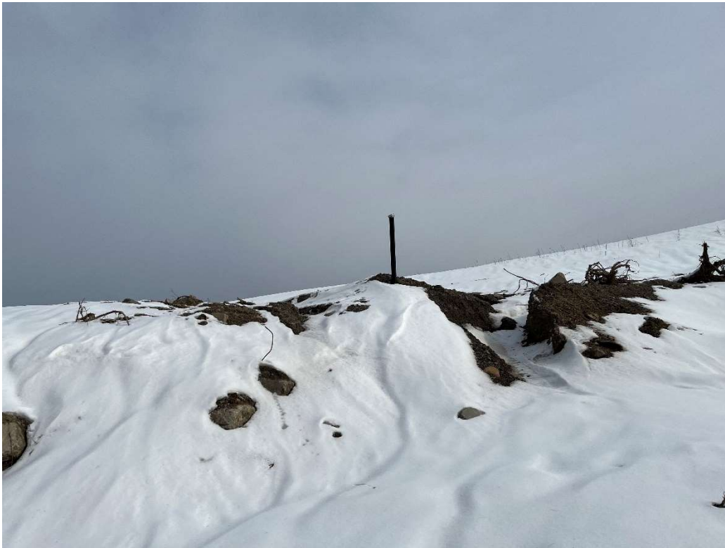
Photo 9 – Grading at monitoring well.
