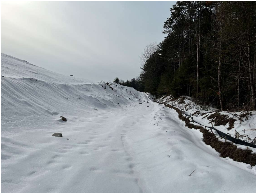
Photo 7 – Representative view of erosion control on the western limits of the Site.
