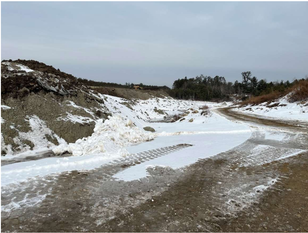
Photo 1 – Eastern slope and access road.
