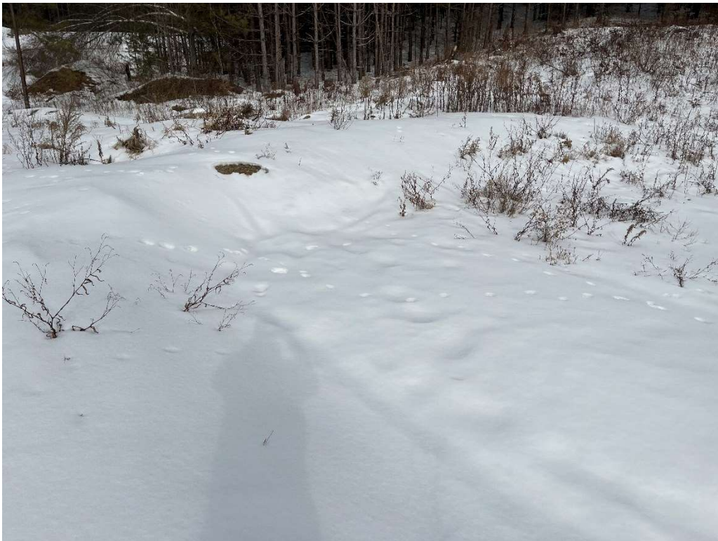
Photo 2 – Temporary stormwater overflow catch basin.
