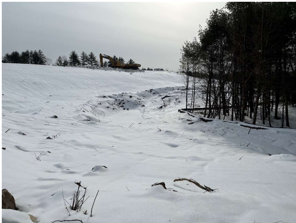
Photo 8 – Southwestern slope and erosion control.
